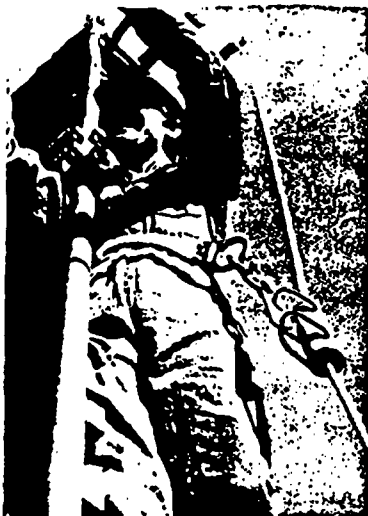
This safety belt and lifeline setup permits the worker to move up and down. The anchoring mechanism will lock instantly in case of fall. (Photo: Research and Trading Corp.)
