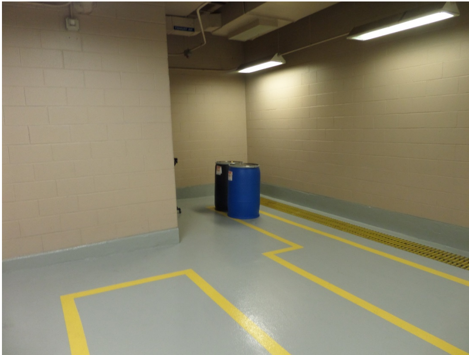
Photograph 17: Partial view of the Flammables Storage Room 115.
