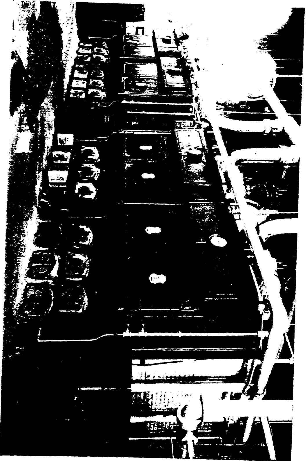
FOUR 302 H. P. HEINE BOILERS, MONOMAC SPINNING CO., LAWRENCE, MASS.
