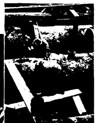
Pouring and calking lead joints in some of New York's 48-in. cast-iron mains. The center view gives an idea of the complexity of New York's underground system
