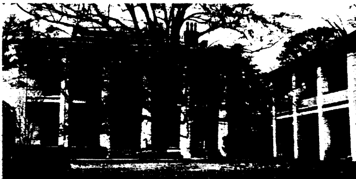
Rear of Melrose, which is one of the few mansions still following the old custom of housing kitchen and servants' quarters in a separate building. at right. White lead is used on both structures
