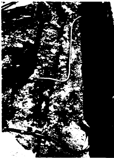
Lead connections joining old lead services at left to a new main in New York. Note goose-necks to provide for movement
