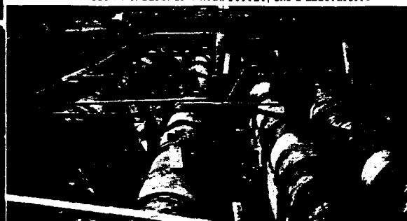
Pouring and calking lead joints in some of New York's 48-in. cast-iron mains. The center view gives an idea of the complexity of New York's underground system
