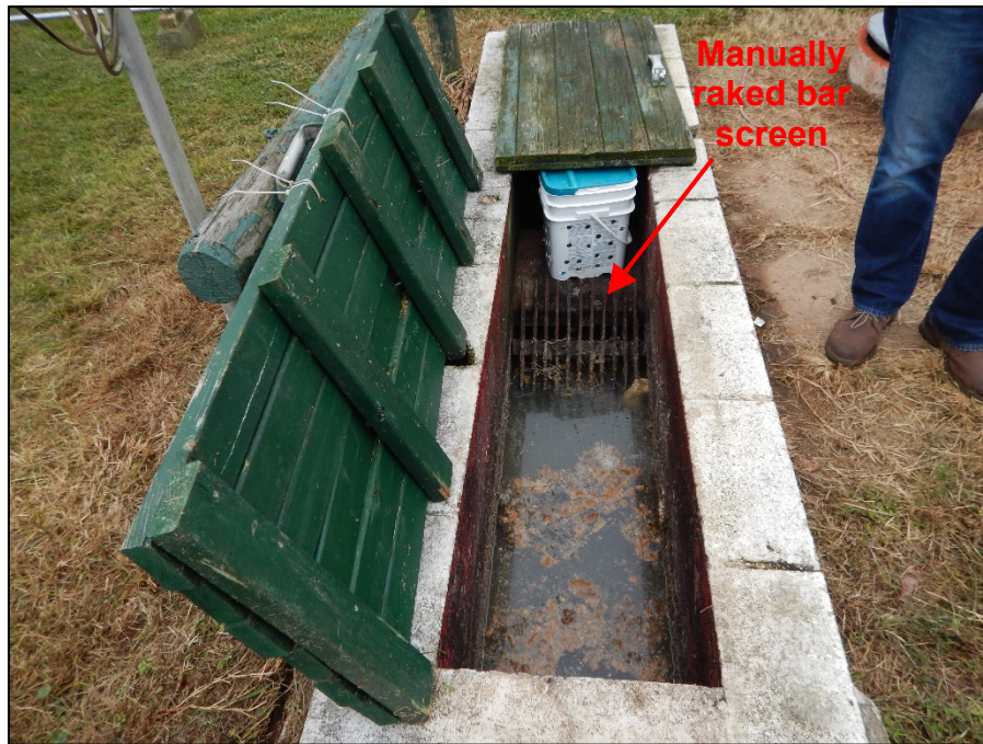
Photograph 3. View of the influent bar screen.
