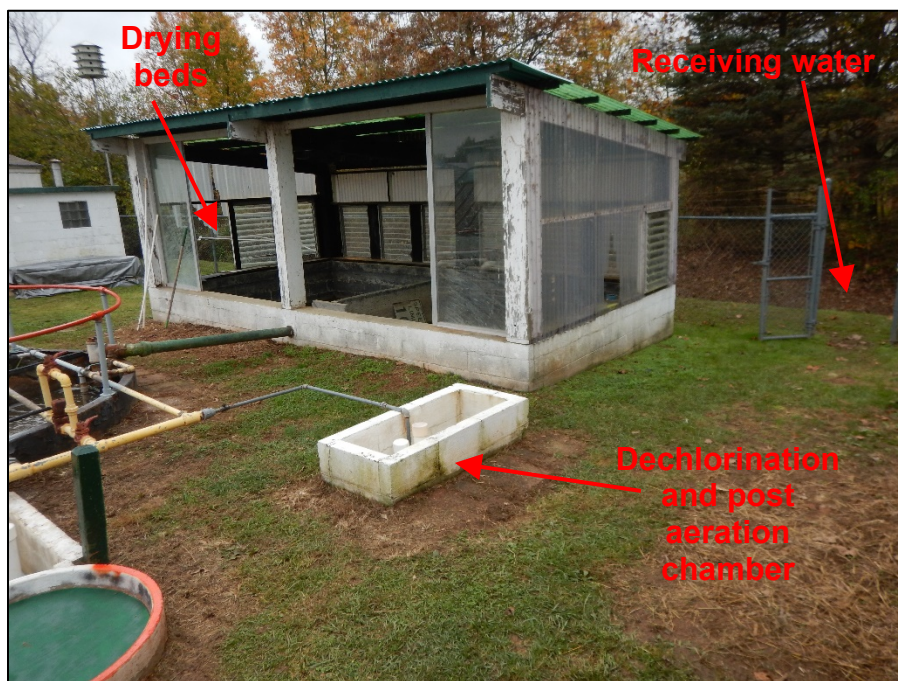
Photograph 16. View, facing southwest, of the out of service drying beds. Also, note the location of the dechlorination and post aeration chamber and receiving water.
