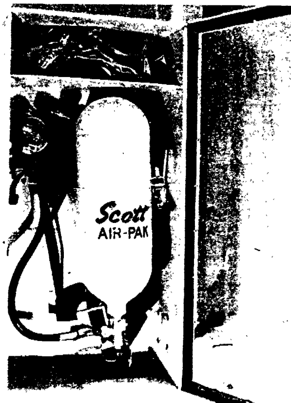
Figure 9-6. Wall-mounted storage cabinet for a SCBA.
