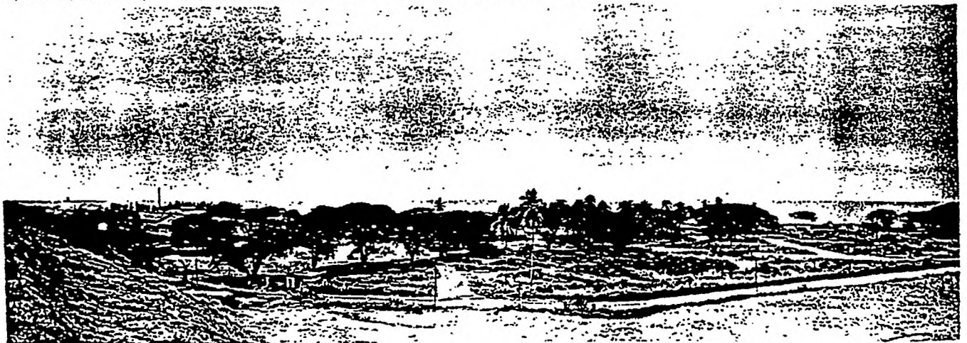
A portion of new steel plant site, Mindanao, Philippines. In foreground, site preparation is under way.
