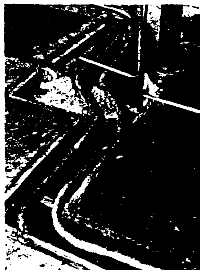
Above, supply line and two return lines, all lead, from hydraulic presses.
