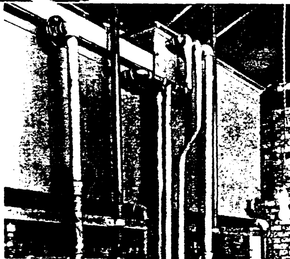
Above, supply line and two return lines, all lead, from hydraulic presses.
