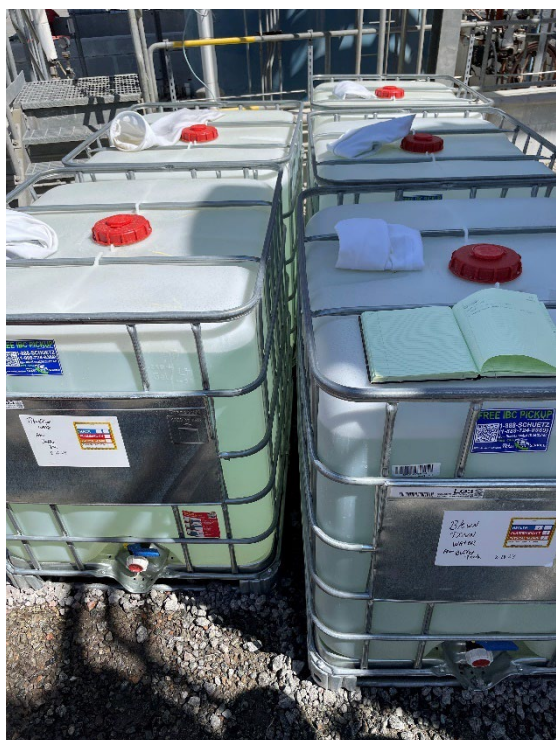
Figure 7: IMG_3250.jpg – Blow down water in totes
