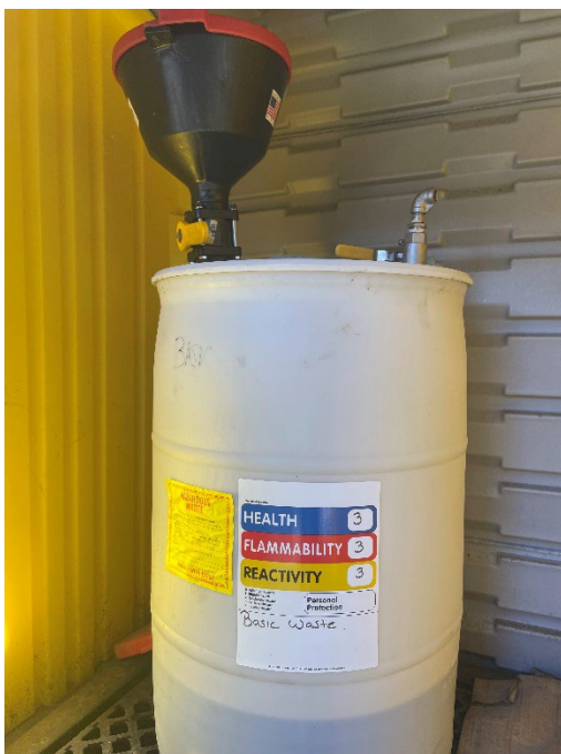
Figure 57: IMG_3309.jpg - North Plant SAA
