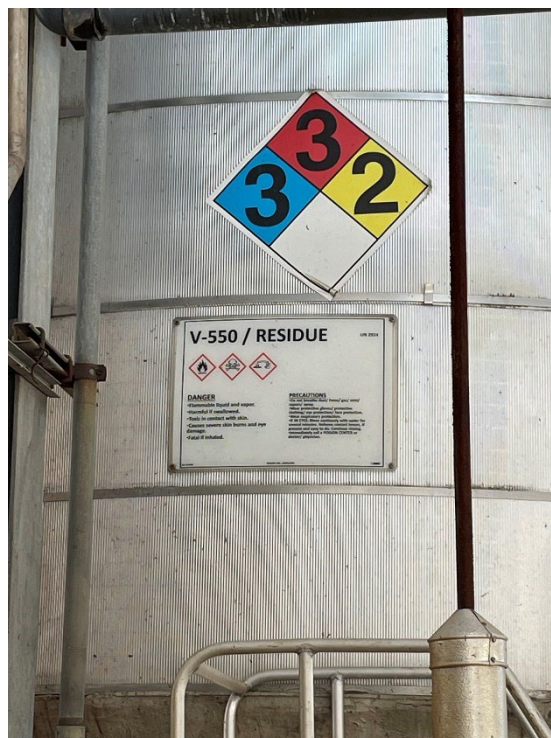
Figure 12: IMG_3255.jpg – Hazardous Waste Tank V-550
