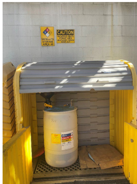
Figure 58: IMG_3310.jpg – North Plant SAA #2
