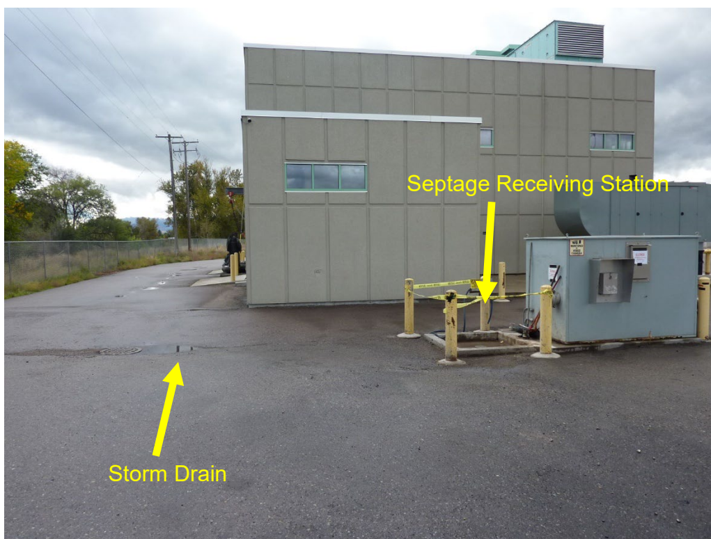
Figure 6 – Missoula Septage Receiving Station
