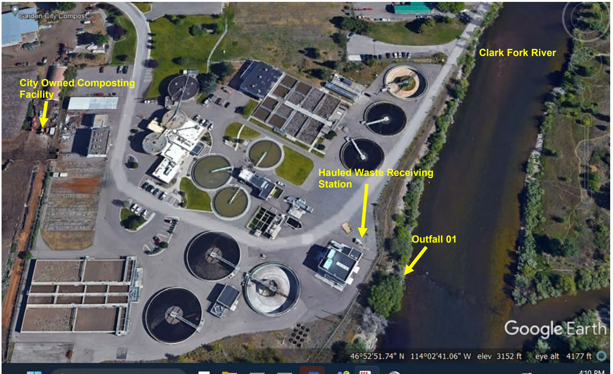
Figure 5 – City of Missoula POTW – Google Earth View
