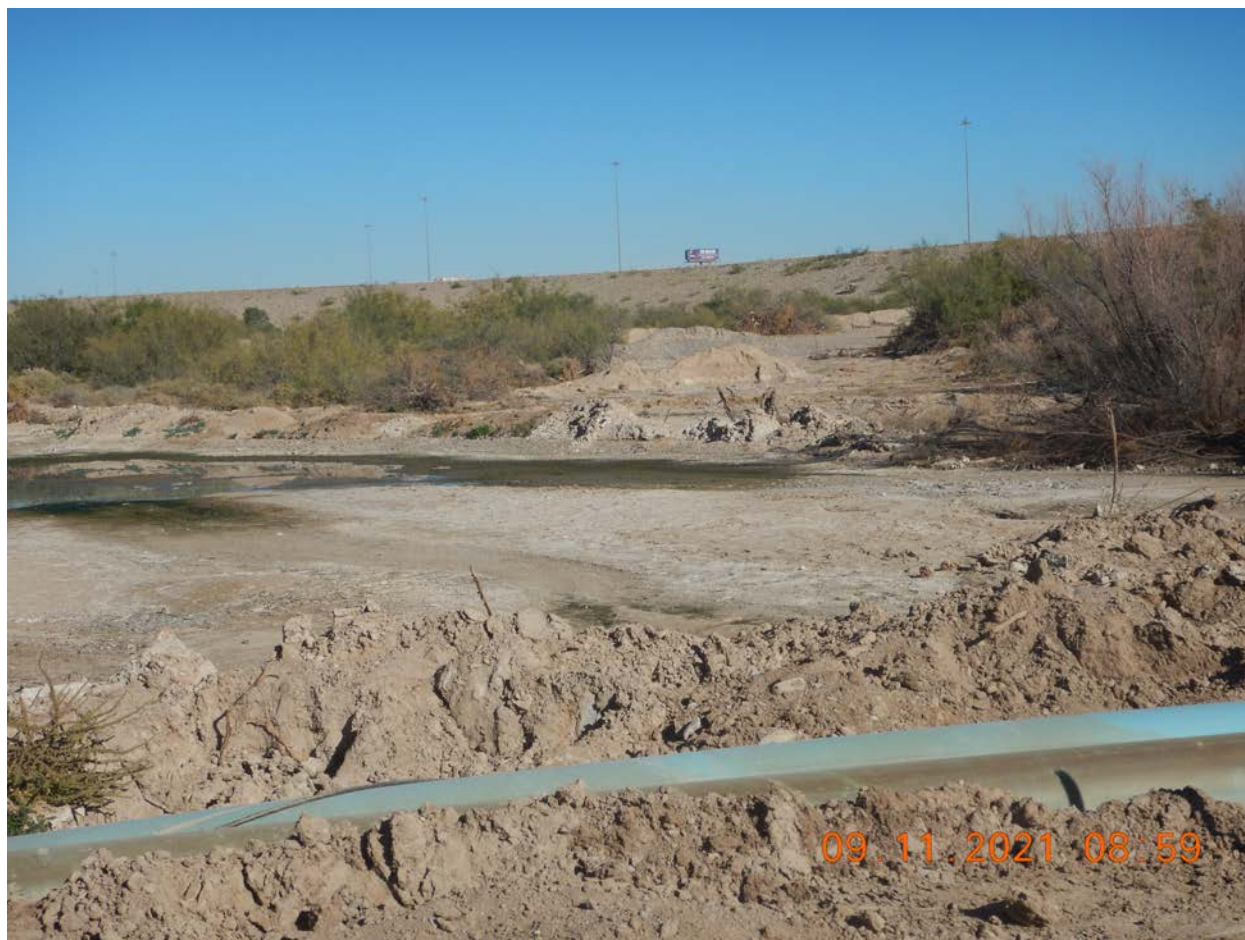
View of earthen berms constructed to contain wastewater flows, prior to placement of temporary above ground piping. Note: the lift station is in the approximate lower right of the photograph. (DSCN2002). Photographed by D. Esparza
