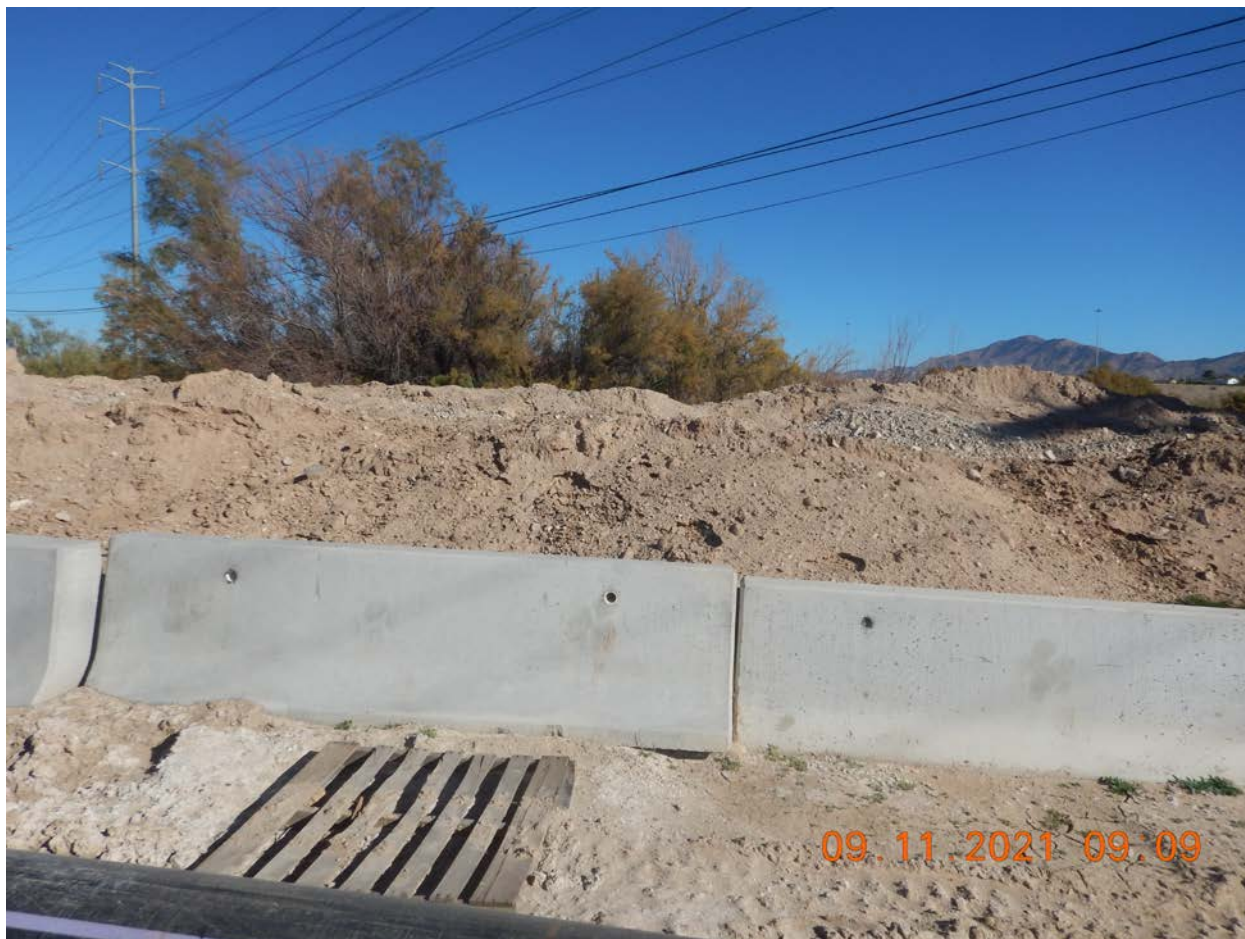
View of the constructed earthen berm and above ground temporary by-pass piping in foreground. Note: concrete barriers typically placed to prevent wash-out. (DSCN2005). Photographed by D. Esparza
