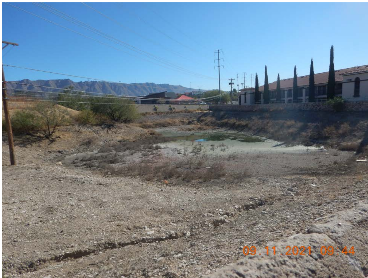
View of retention pond located along the approximate southeast side of Doniphan Park Circle. (DSCN2010). Photographed by D. Esparza
