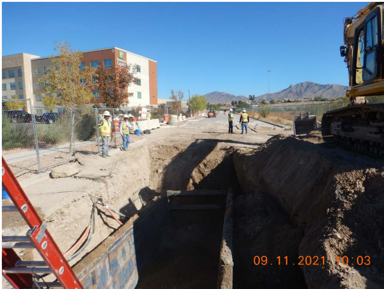
View of open excavation in the vicinity of the new alignment utilizing an existing abandoned 54-inch water line and a "slip line method" of placement to hasten replacement. (DSCN2024). Photographed by D. Esparza
