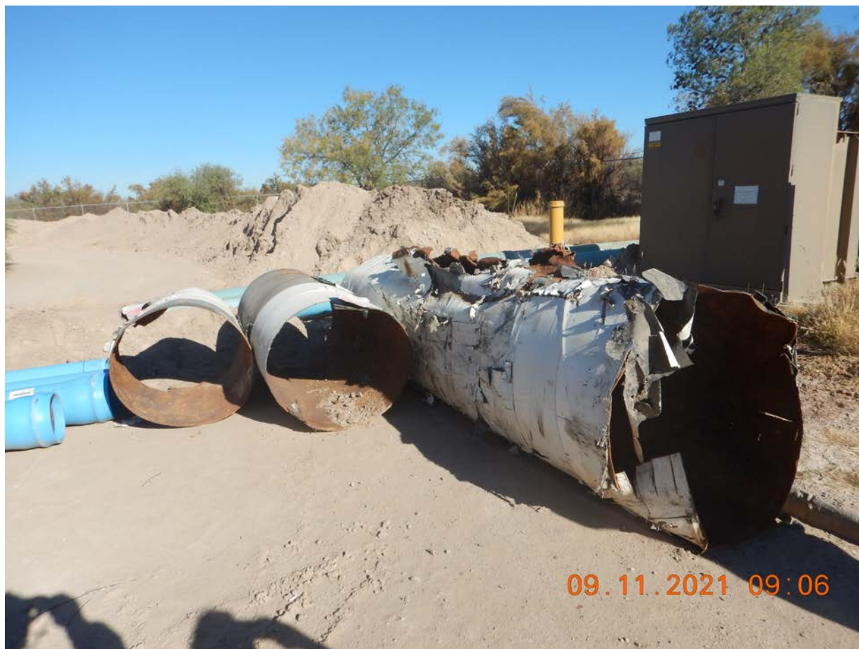
Previously existing collection lines staged in proximity of Frontera Lift Station awaiting forensic analysis. (DSCN2003) Photographed by D. Esparza
