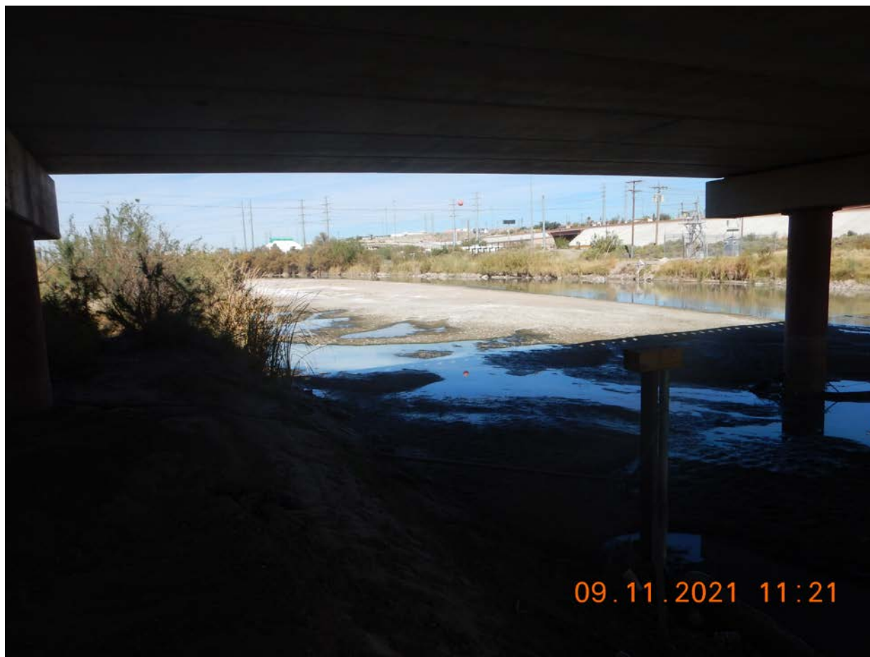
View beneath the Courchesne Bridge looking towards the approximate north. (DSCN2048) Photographed by D. Esparza
