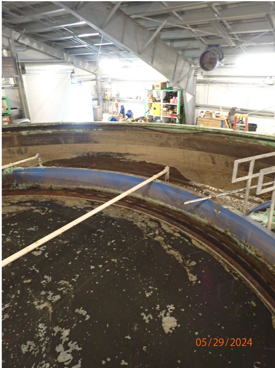
Photo 3 - Same clarifier from a different angle
