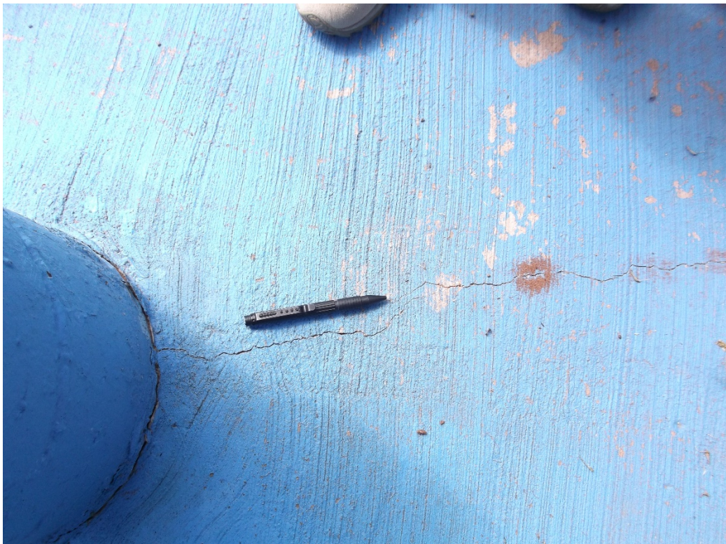
Photo 8. Concrete pad at Mares and Grizzle wells location
