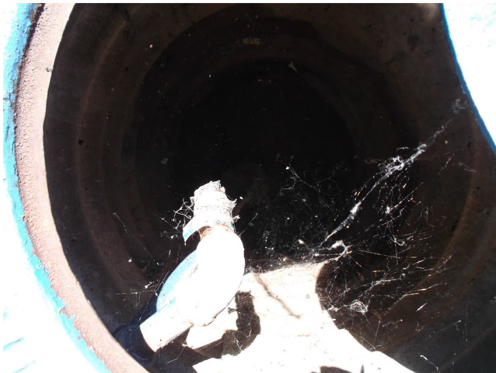
Photo #10. Screen on the air relief valve for Grizzle well.
