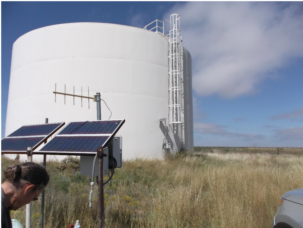
Photo 2. Grizzle Tank area overrun with vegetation, making it difficult (and potentially hazardous) to observe problems and perform maintenance
