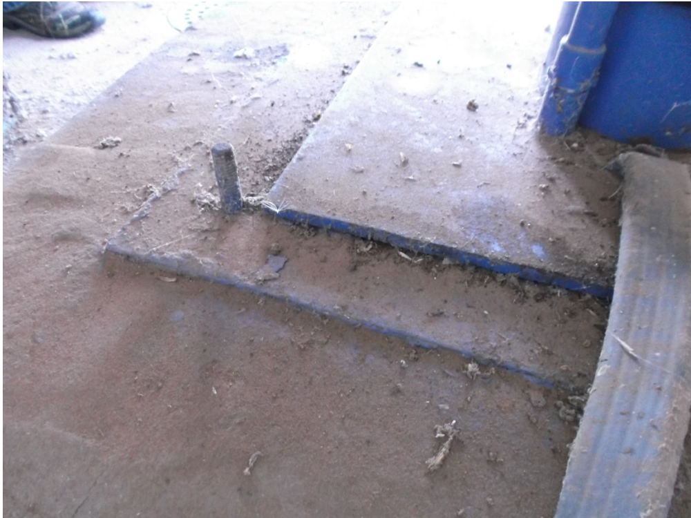
Photo #11. Gap in the well plate at the Grizzle well
