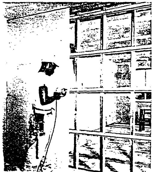
STEP 2—SHEETROCK gypsum wallboard is attached with Type "S" drywall screws, 12 in. o.c. (below). Note top channel 6 in. below ceiling line, bottom channel 24 in. from floor; scrap \frac{1}{2} -in. wallboard forms base filler strip.
