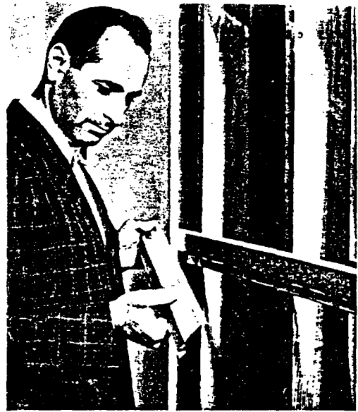
NO MORE "PARTY" in this party wall. New USG resilient channel makes drywall a better sound barrier, say progressive builders who have used it.
