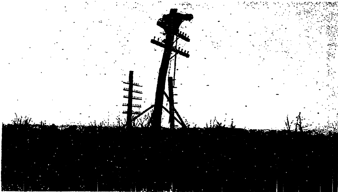
Slide No. 3. Correct method of removing cross-arms from defective pole.
