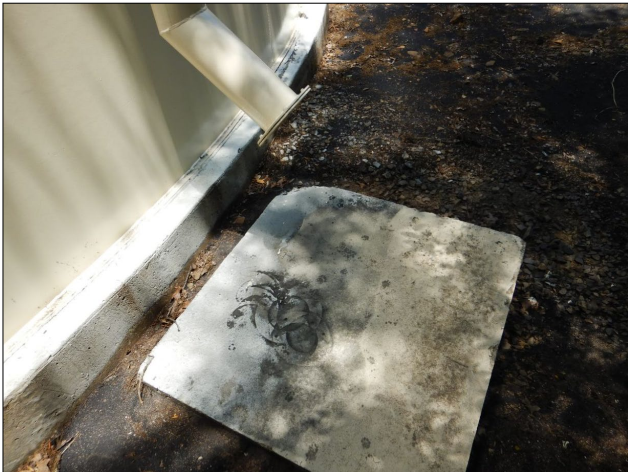
Photograph 6. Splash Pad, Gum Log Storage Tank View of the splash pad beneath the overflow line at one of the Gum Log Storage Tanks. The second tank contained a splash pad that was similar to this one.
