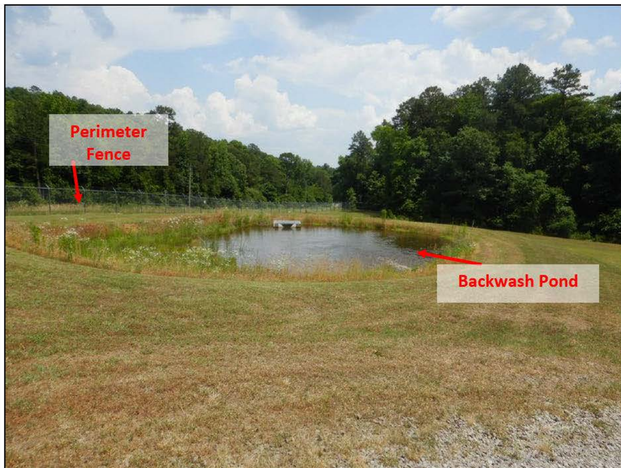
Photograph 11. Perimeter Fence, Hector WTP View of the locked perimeter fence with barbed wire that surrounds the Hector WTP property. Also pictured is the pond that filter backwash product is sent to.
