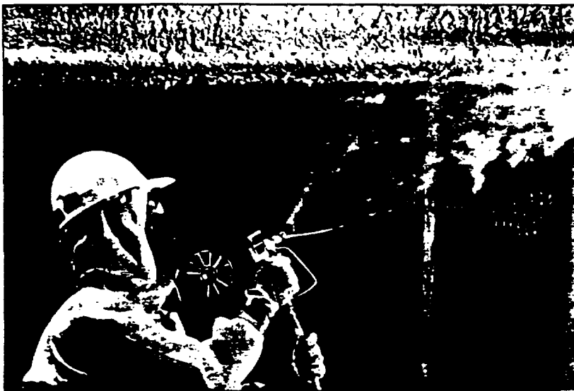
Well protected, well trained technician applying wetting agent to asbestos prior to removal.
