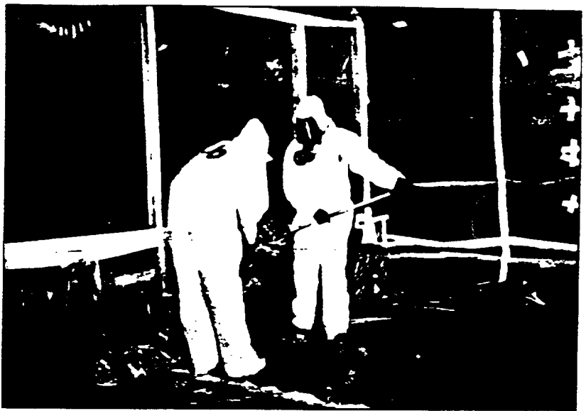
Cleanup of asbestos debris. All work is carried out within containment to prevent the release of asbestos fibers to the surrounding environment.
