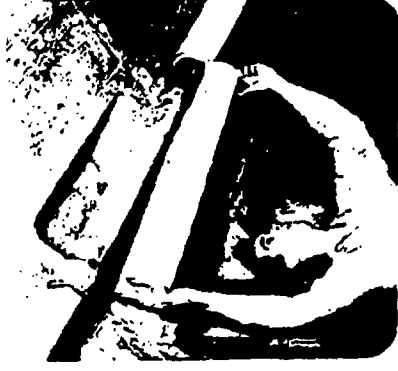
The single jacket on Flame-Safe means that there is no need for a separate vapor barrier. The single layer is sufficient to provide the required protection.
