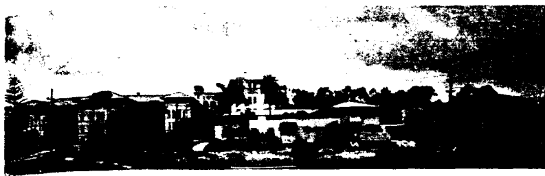
San Diego County Hospital. The old buildings at the left have lead plumbing that has never given trouble, while the new buildings, at right, have had trouble with newer plumbing that is not lead
