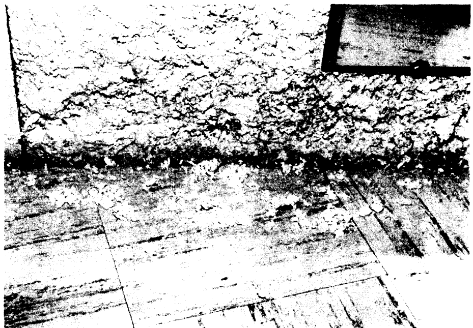
Asbestos-containing wall insulation deteriorated and falling to the floor.
