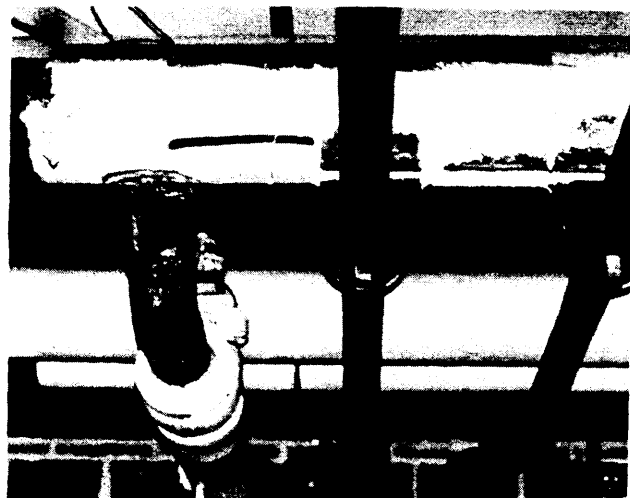
Preformed, asbestos/magnesia, pipe wrapping covered by a protective jacket.
