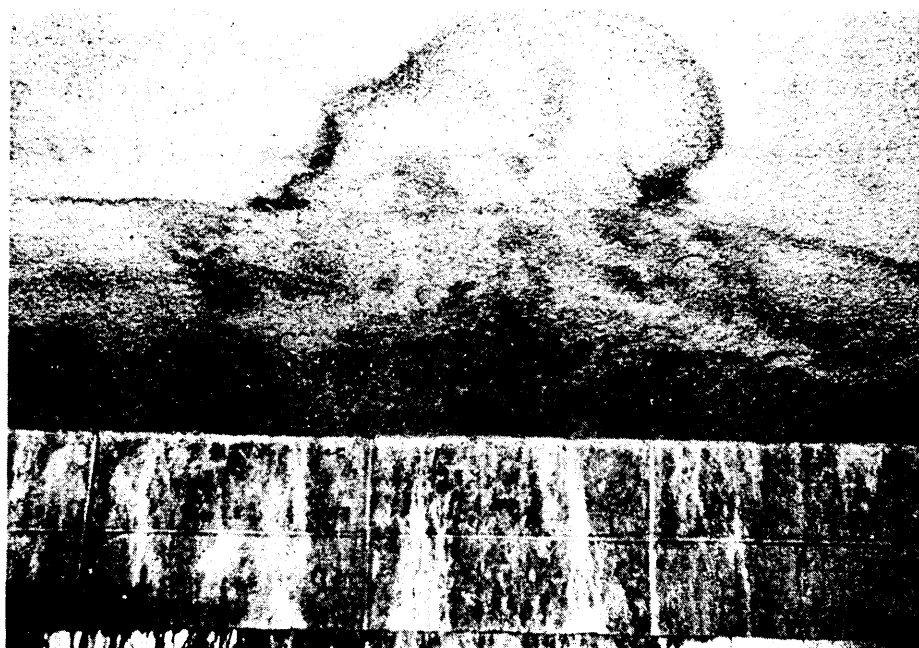
Water has leached asbestos fibers from the acoustical plaster ceiling, carried these fibers down the wall and evaporated leaving a deposit of asbestos fibers on the wall.
