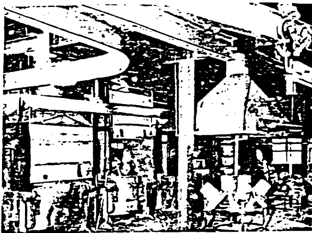
Fig. 2—Partially-enclosing hoods have been fitted to the tilting furnaces shown at the left of photograph.
