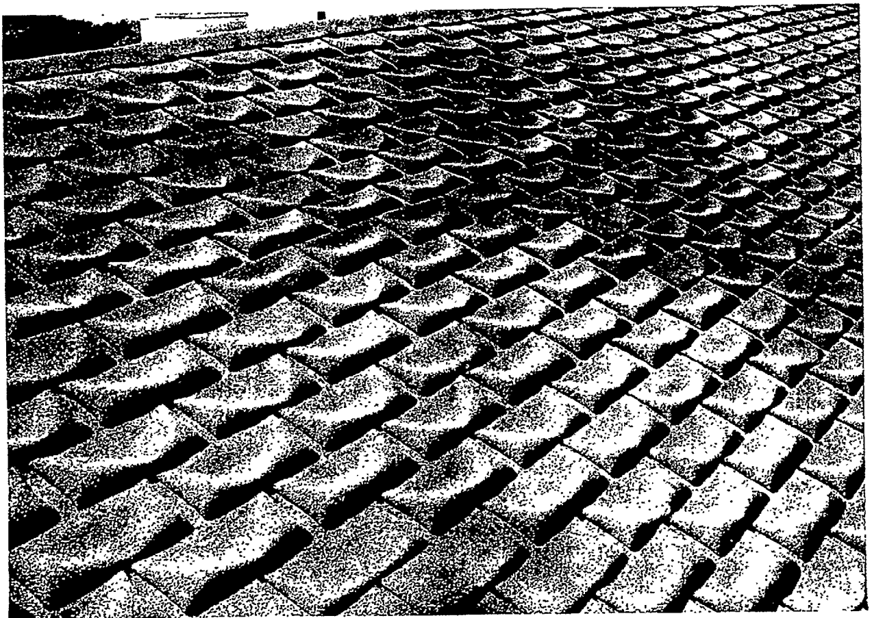
Figure 26. Clawed asphalt strip shingles.
