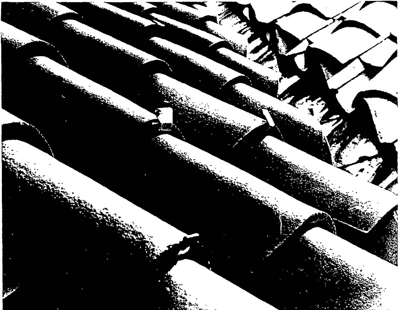
Figure 38. Replaced tiles fastened in place with metal strips.
