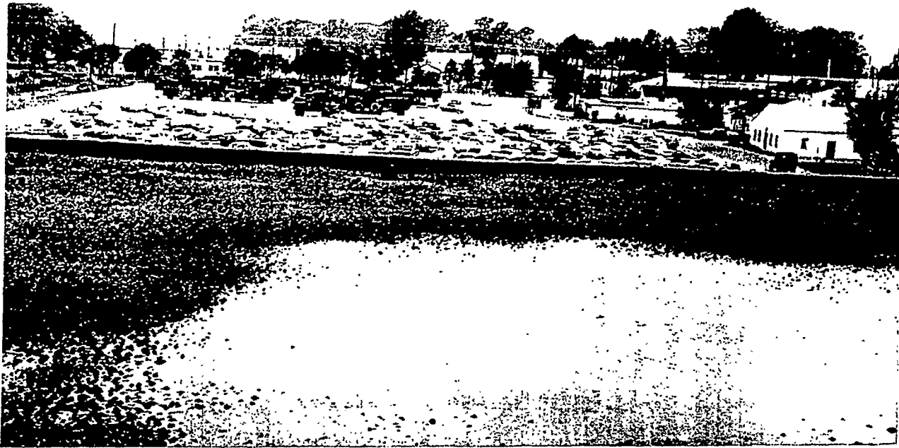
Figure 52. Drain not located in low area—ponding sometimes caused by structural defect.
