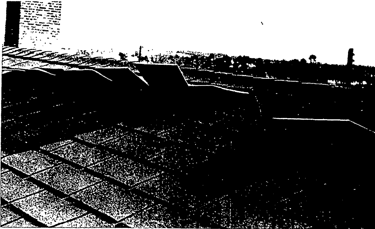
Figure 6. Action of wind on shingles nailed too high—can be eliminated by proper nailing and using wind-resistant shingles.
