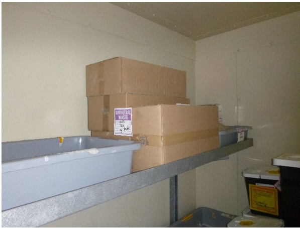
Photograph 39: CAA waste universal lamps.
