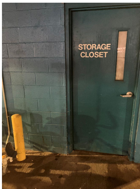
Photograph 49: Garage Storage Closet for Universal Waste Lamps.
