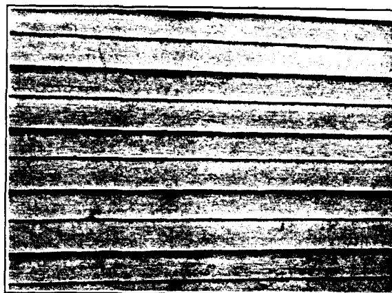
Detail of white lead paint on siding after seven years' exposure. Wood still well protected and surface perfect for repainting.
