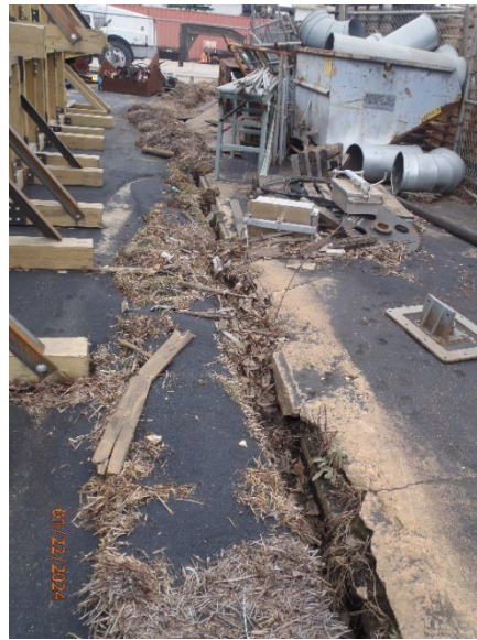
Picture 8 – External Blast Media – non-hazardous black beauty media released to storm water drain
