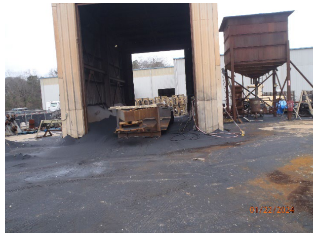
Picture 4 – External Blast Media – non-hazardous black beauty media released to ground
