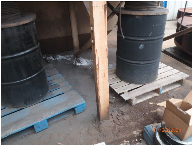
Picture 2 – Internal Blast Booth SAA –baghouse dust released to the ground
