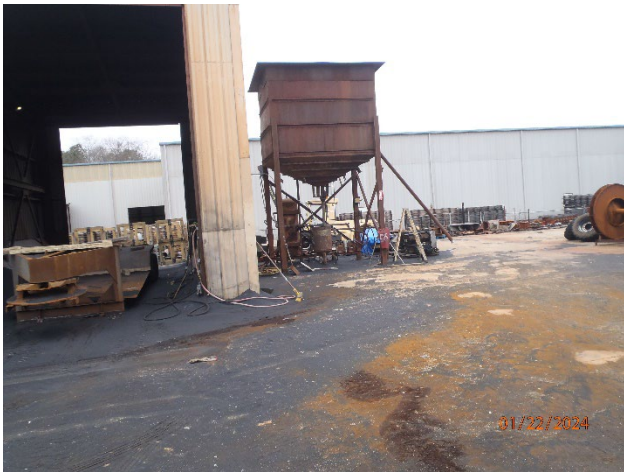
Picture 6 – External Blast Media – non-hazardous black beauty media released to ground
