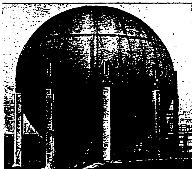
Pyroscat applied to columns of spherical tank
