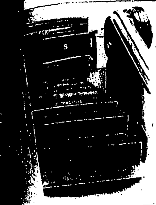
10 Old-type smooth-tread-step moving stairways required a shunt S at the landings to guide the passengers on and off
