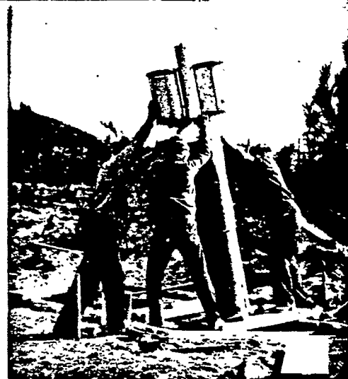
• INSTALLING gasoline tank at Forest Service Remount Depot.
