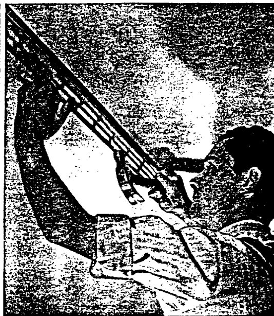
SECOND, securely attach the L-shaped metal ceiling runner. Center the top flange over the center line of base. The three horizontal slots allow for minor variations in ceiling height.
