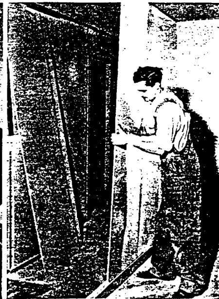
THIRD, place bottom edge of long length ROCKLATH plaster base in set grouted base section. Top edge against the vertical flange of ceiling runner. Position against V-edge of preceding
