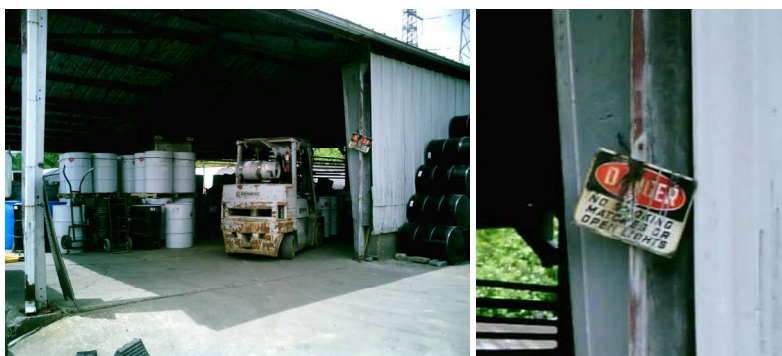
Figure 1: Photograph 8 – Flammable Danger sign in Dock Area
