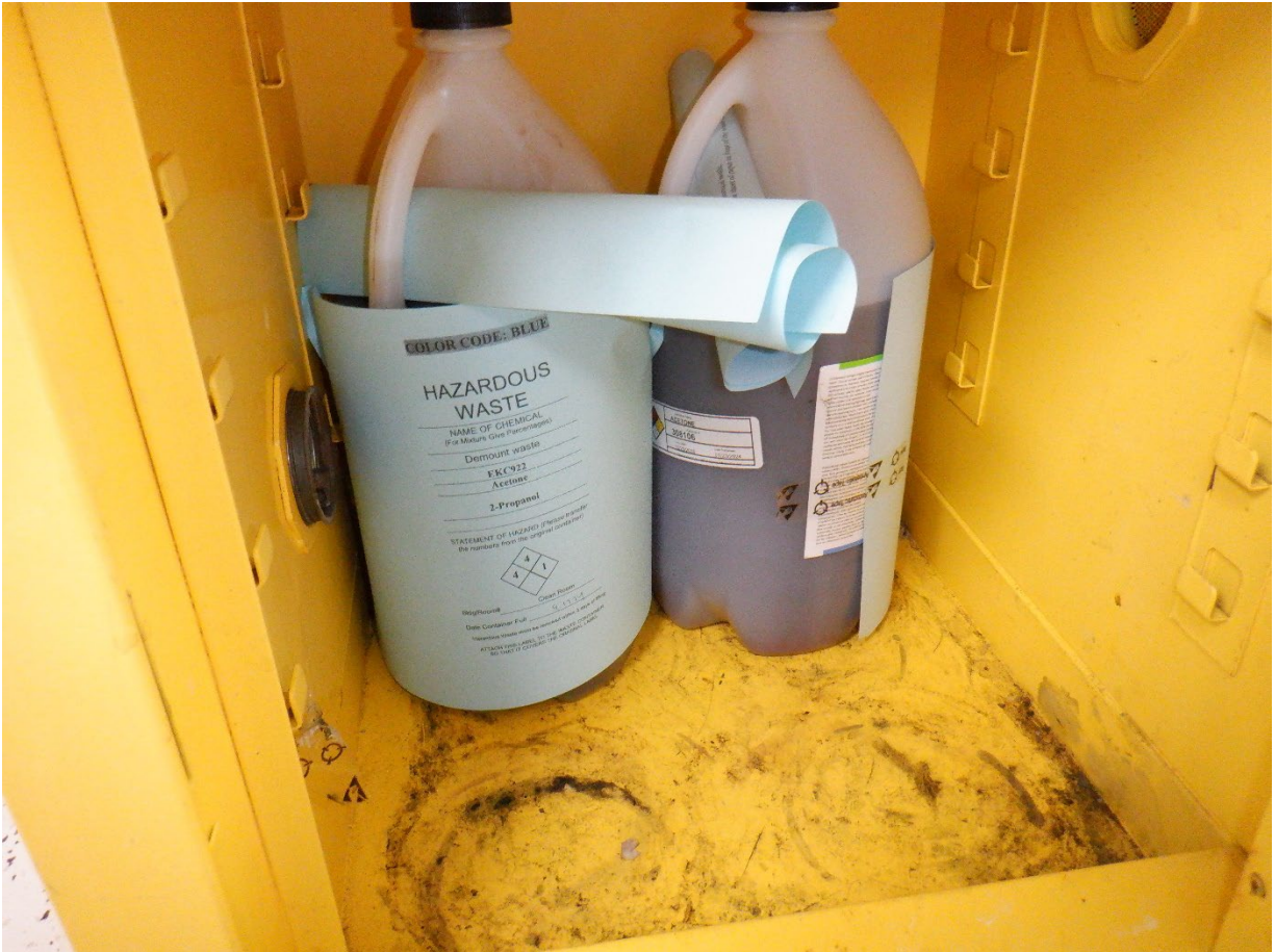
(Figure 1: Showing chemicals inside of the ignitable cabinet)
