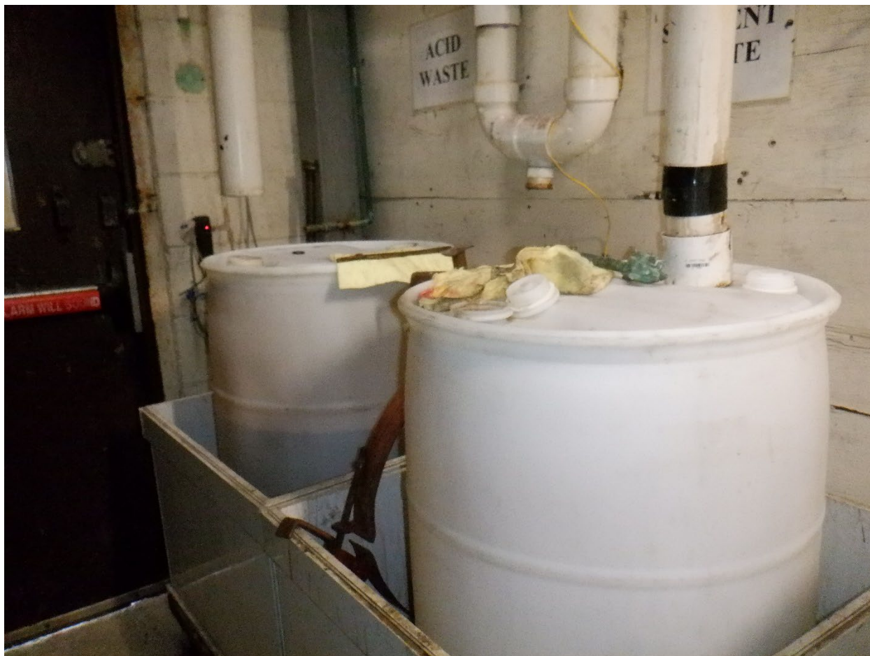
(Figure 11: Showing hazardous waste located in the Central Storage Area with that are open and not labeled with the words hazardous waste or have a date)
