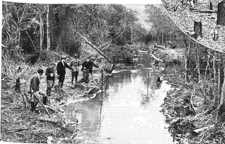
Above—This is how the swamp jungle looked after preliminary clearing had been completed. All underbrush and branches were moved away and the stumps shown here were loaded with extra charges of dynamite.
