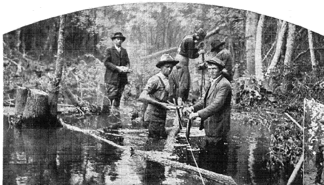
The line of holes for the Moultrie ditch blast often led through pools of muck and water as shown above. Right—a dynamite storage house near the scene of the blasting
