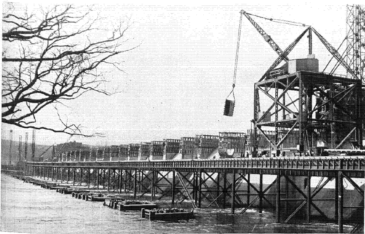
The downstream face of the dam, showing the runway over which cranes and supplies are brought to the scene of operation. One of the traveling giants may be seen in action in this photograph
