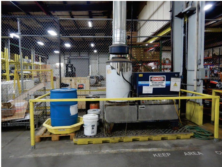
Photograph 2: View of the parts washer and containment area for cleaners used in the washing stage. The black drum at the rear of photo is the coil cleaner. The white bucket in front of the photo is the new caustic cleaning solution that replaced the phosphoric acid cleaner.
