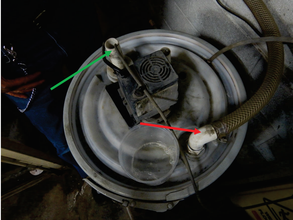
Photograph 5: A view of the top of the final discharge tank. The red arrow identifies the pipe used to convey wastewater from the final sump into the drum. The green arrow identifies the sample point.
