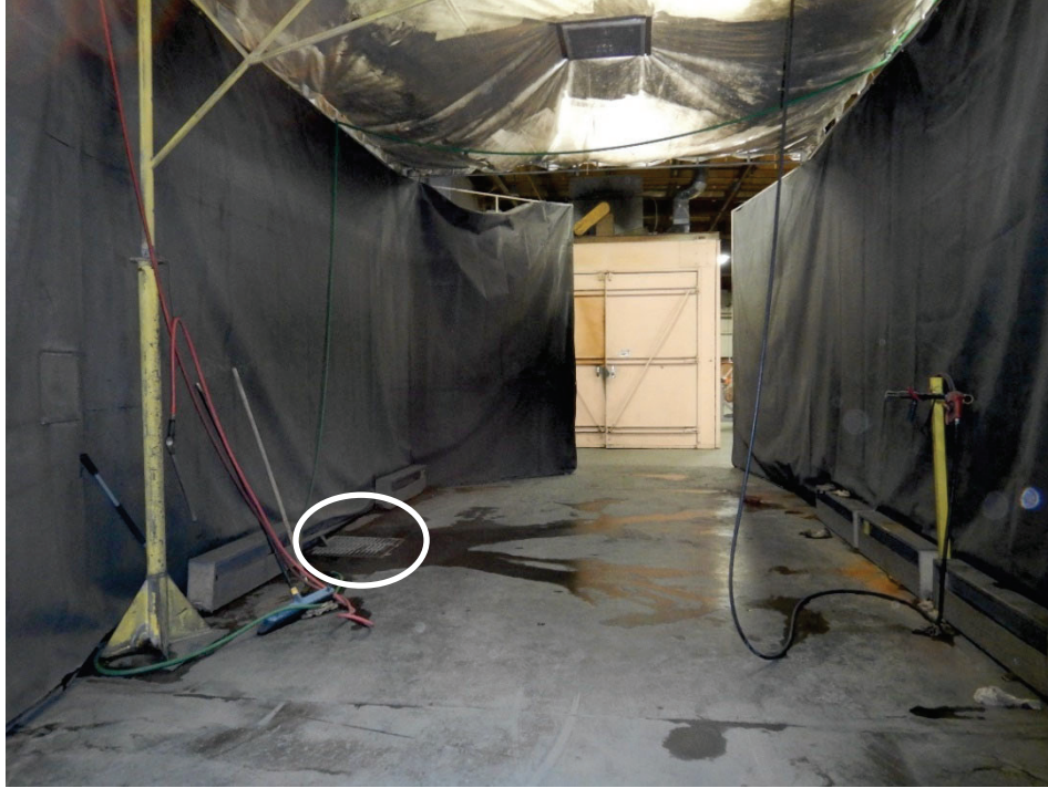
Photograph 1: View of the facility's spray booth. The sump pit (circled) is pumped to the final discharge tank.
