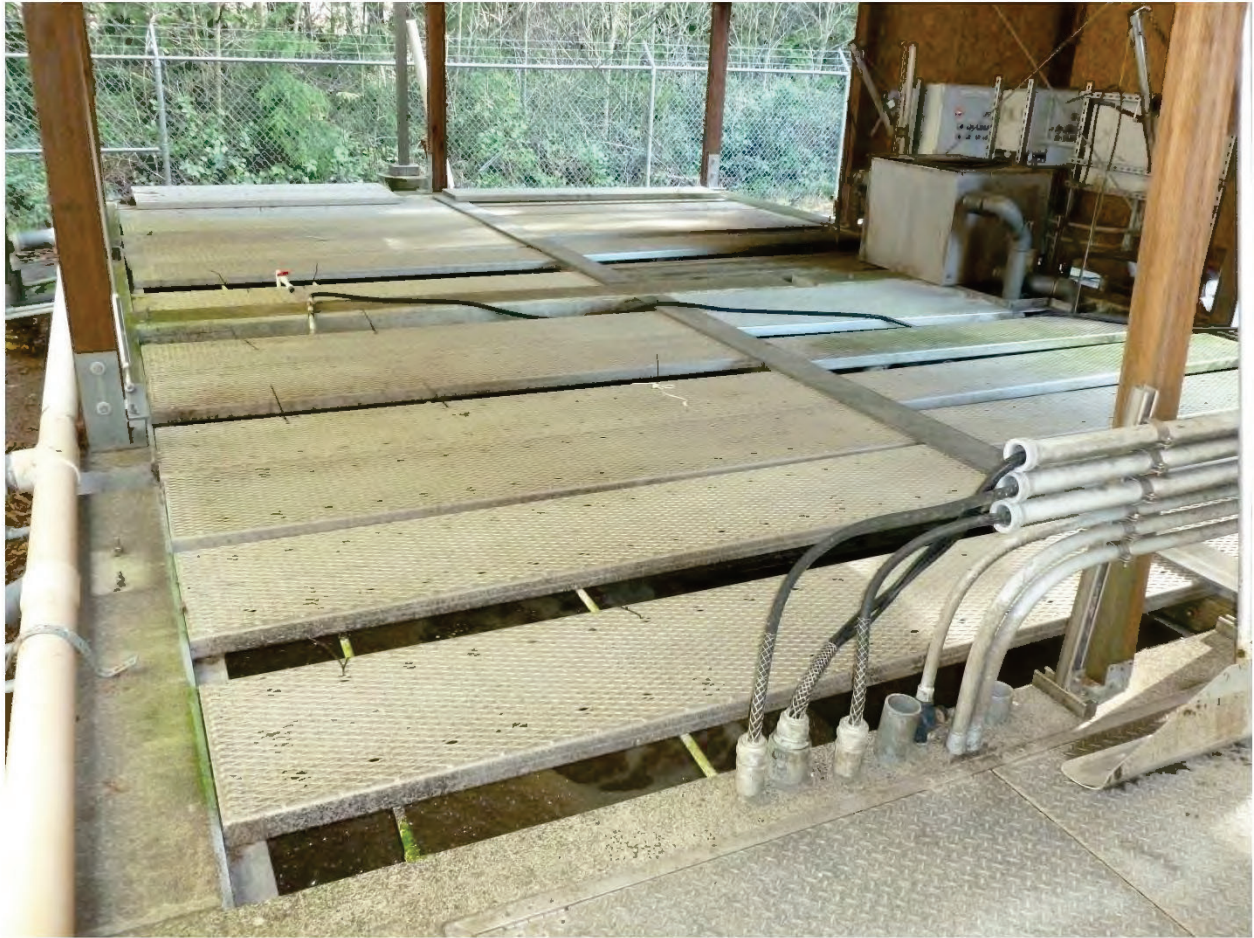
Photo 3 / P1000652 – Deck Planks
