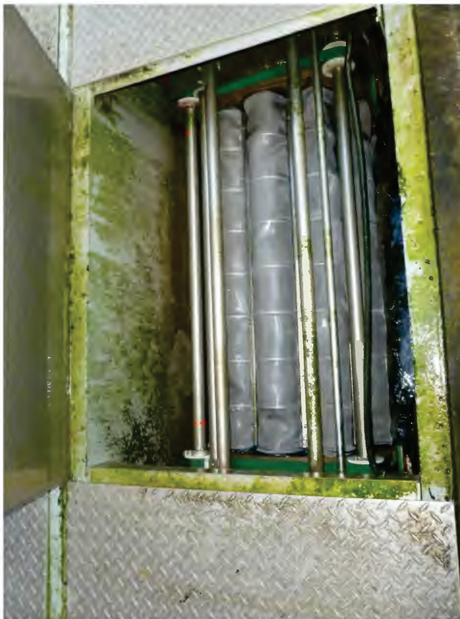
Photo 5 / P1000656 – Microfilter Drums
