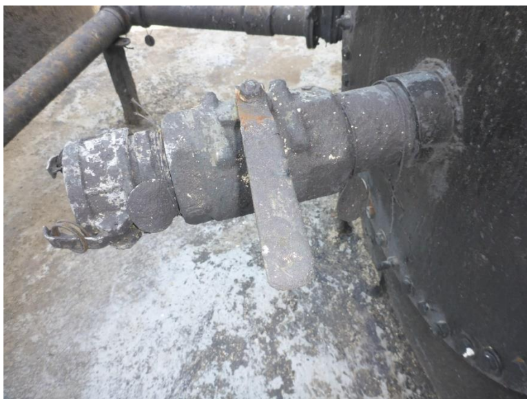
Photo 18: Tags associated with Tank 1736B which were not legible.
