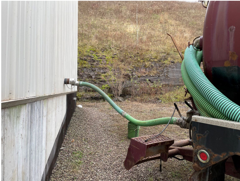
Photo #3. Pretreated effluent is transported by the septic hauler to the POTW for treatment.
