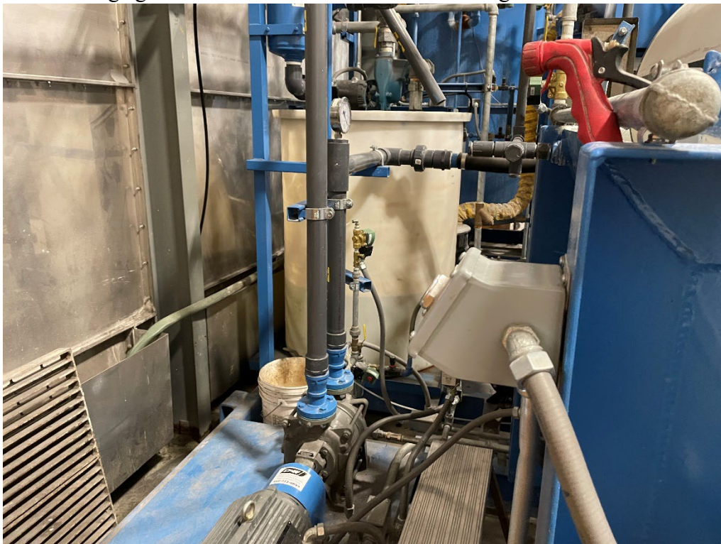
Photo #6. Defoaming agent is added to the filtrate in the holding tank.
