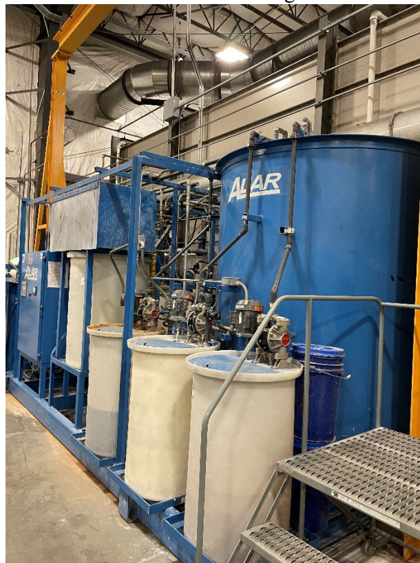
Photo #4. Generated process wash water is treated through the Alar Waste Treatment System.
