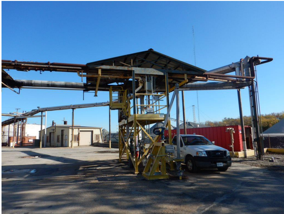
Photograph 4. (DSCN2202) View, facing north, of the Facility truck rack located in the middle of the Facility.
