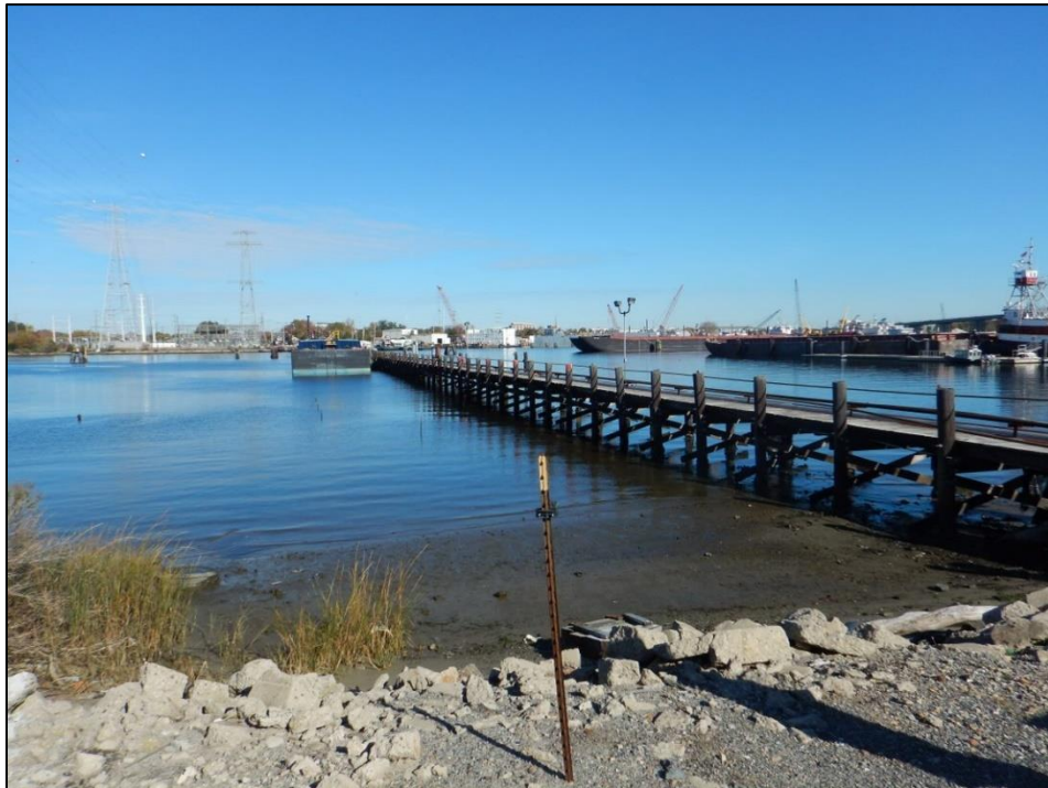
Photograph 10. (DSCN2216) Closer view of the Eastern Branch Elizabeth River and Facility loading dock, as shown in Photograph 9.
