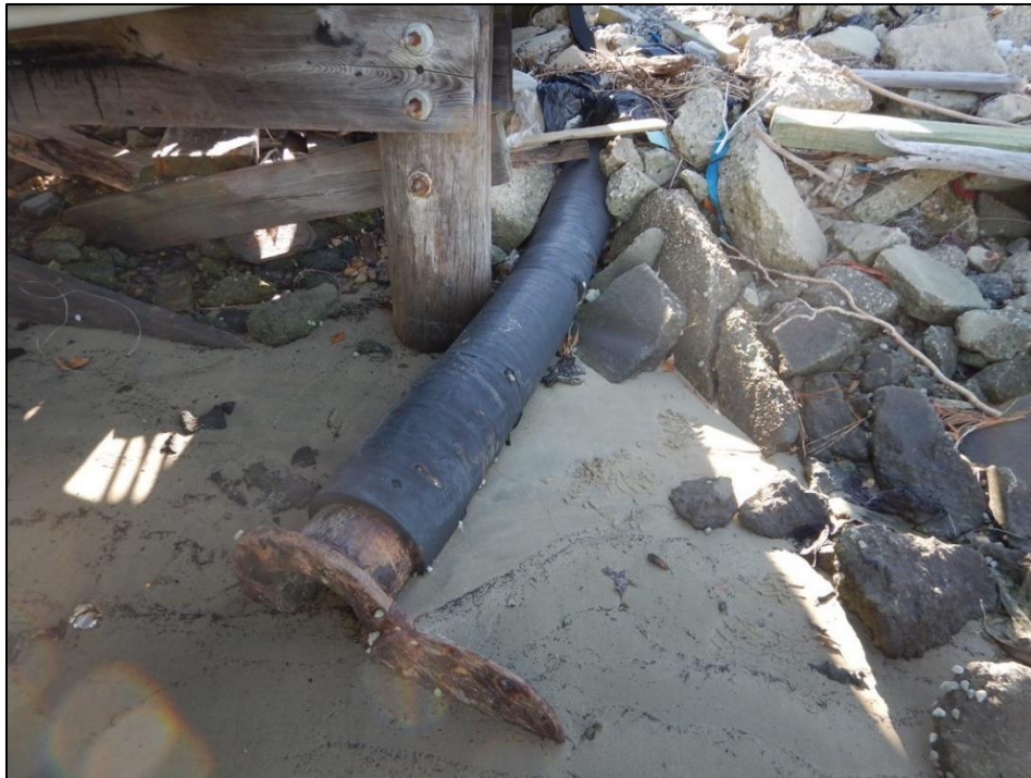
Photograph 13. (DSCN2219) View, facing south, of the outlet pipe for Outfall 001.
