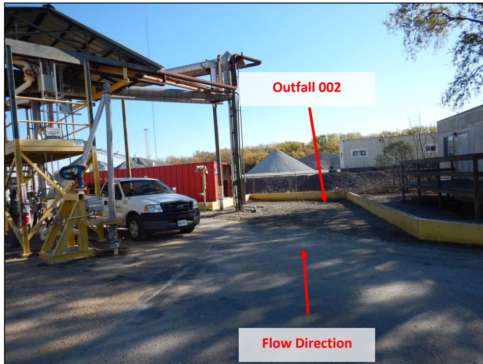
Photograph 5. (DSCN2203) View, facing northeast, of the Facility truck rack as shown in Photograph 4. Note the proximity to Outfall 002.
