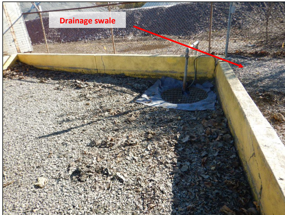
Photograph 1. (DSCN2196) View, facing east, of Outfall 002 located adjacent to the Facility truck rack. This outfall receives sheet flow from the adjacent parking lot and truck rack areas. Flow from this outfall is manually pumped to the drainage swale identified in the photograph.
