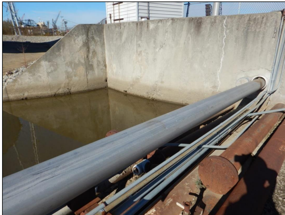
Photograph 8. (DSCN2212) Closer view of the collection area for Outfall 001, as shown in Photograph 7.
