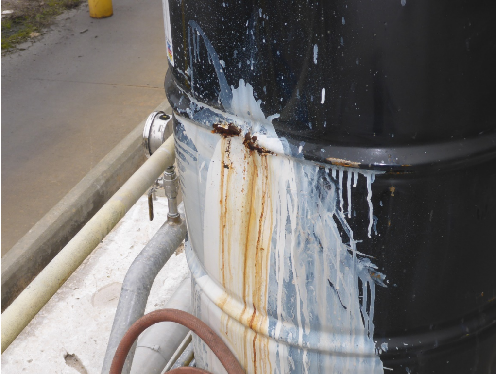
Photo 27: Damage to the 55-gallon drum observed on a secondary containment pallet on the loading dock outside of the hazardous waste CAA. The drum was labeled D001 / F003 / F005 hazardous waste flammable liquid (acetone / toluene) and identified with a flammable liquid DOT hazard placard. The drum was dated 10/07/2020, and the secondary containment unit was full of liquid. Mr. Lucas explained that the drum was hit with a forklift during loading activities, which caused it to leak. Because the leaking drum could not be loaded onto the truck for transport off-site, it was moved out to this portable secondary containment unit.
