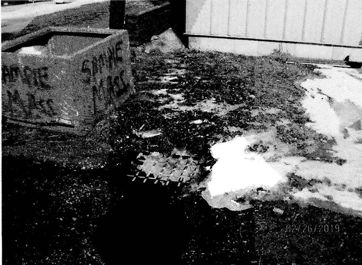
Photo No. 6 Storm Drain
