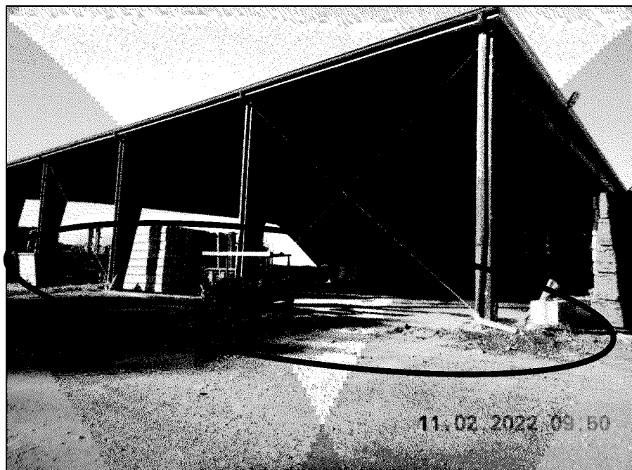
Photograph 4. View, facing west, of the drip pad on the east side of the treatment plant, circled in red, where treated lumber dries before it is moved in the north staging area.
