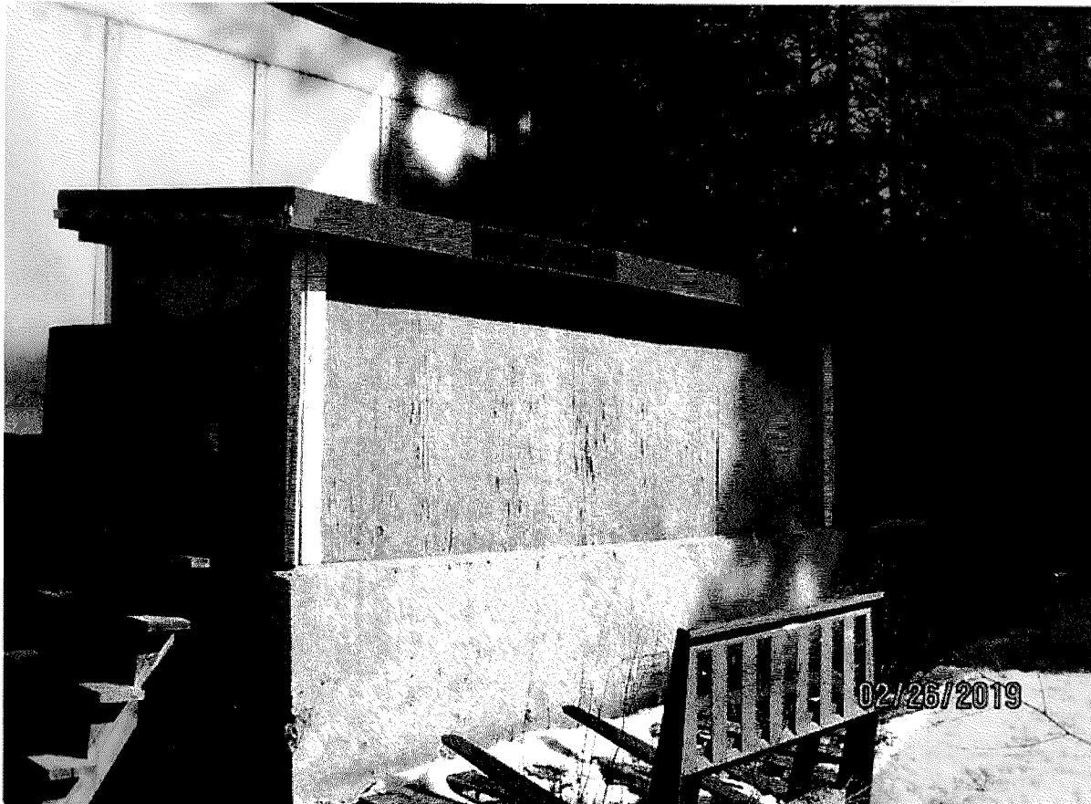
Photo No. 4 Diesel Fuel Tank by Kiln Building
