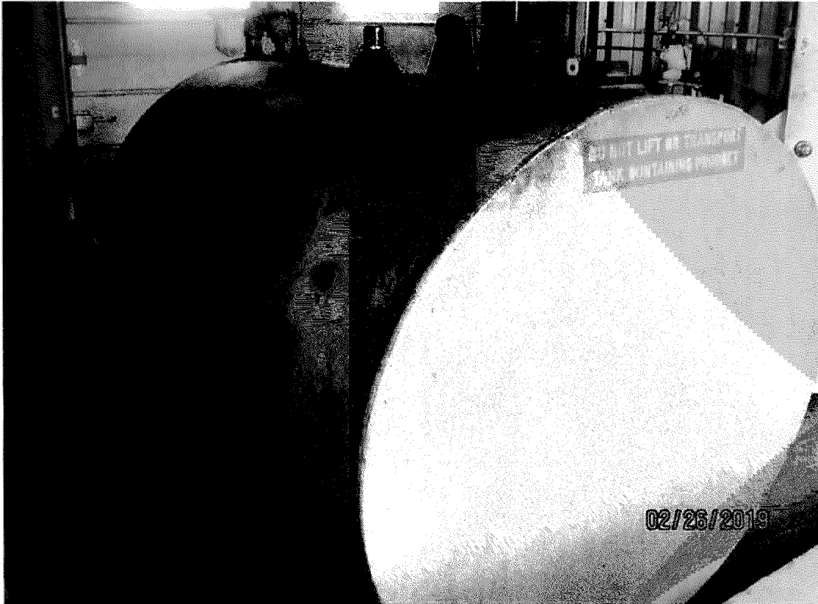
Photo No. 5 Diesel Fuel Tank in Boiler Room
