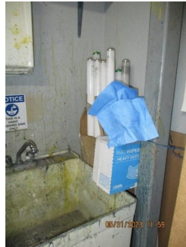
Photo 34: Ten (10) spent fluorescent bulbs in an open container, not labeled with the words "Universal Waste", or marked with an accumulation start date.
