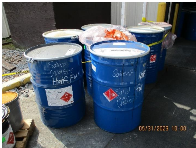
Photo 8: 55-gallon container of solvent waste, no hazardous waste label and no start accumulation date.
