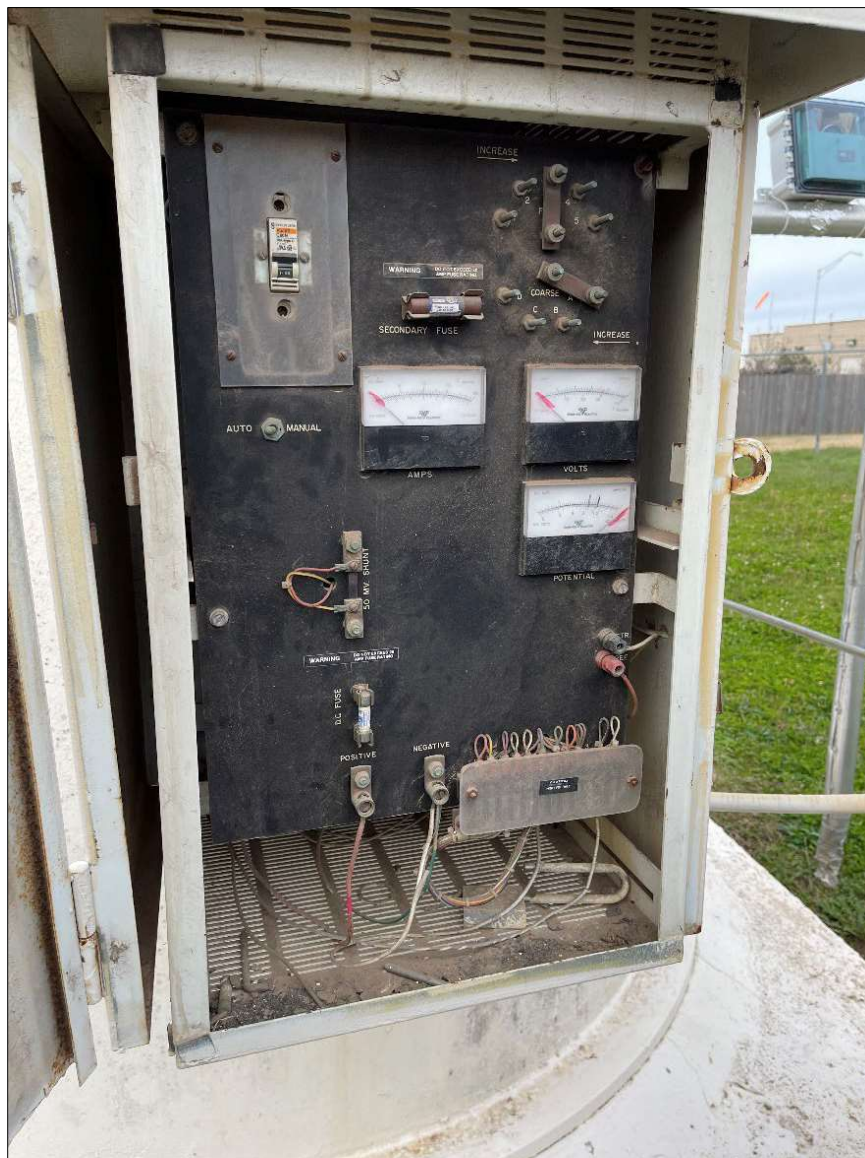
Photograph 16. A Tower South IMG_3112.jpeg
