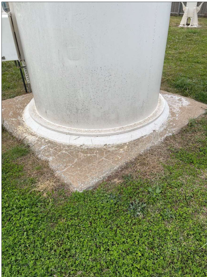
Photograph 12. A Tower North IMG_3107.jpeg
