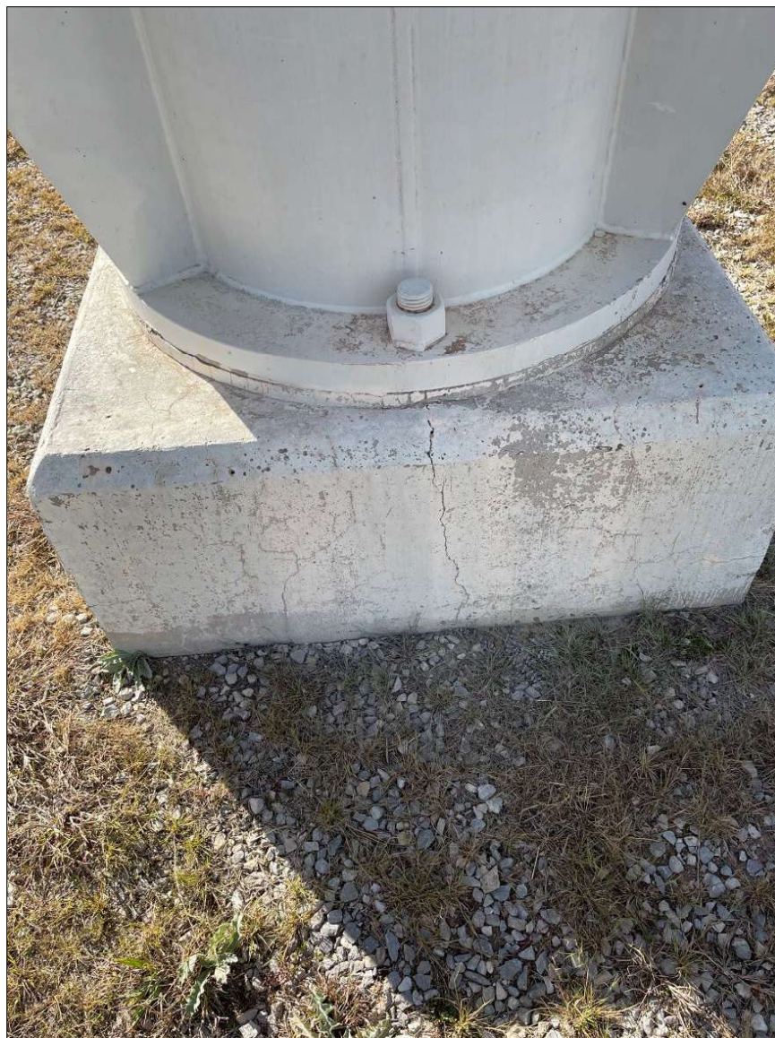
Photograph 13. Navy Tower IMG_3136.jpeg
