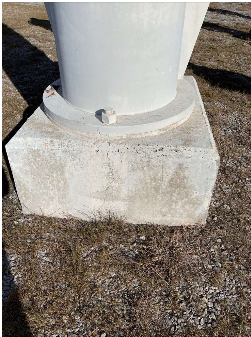
Photograph 14. Navy Tower IMG_3137.jpeg
