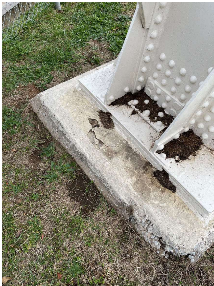
Photograph 11. A Tower North IMG_3106.jpeg
