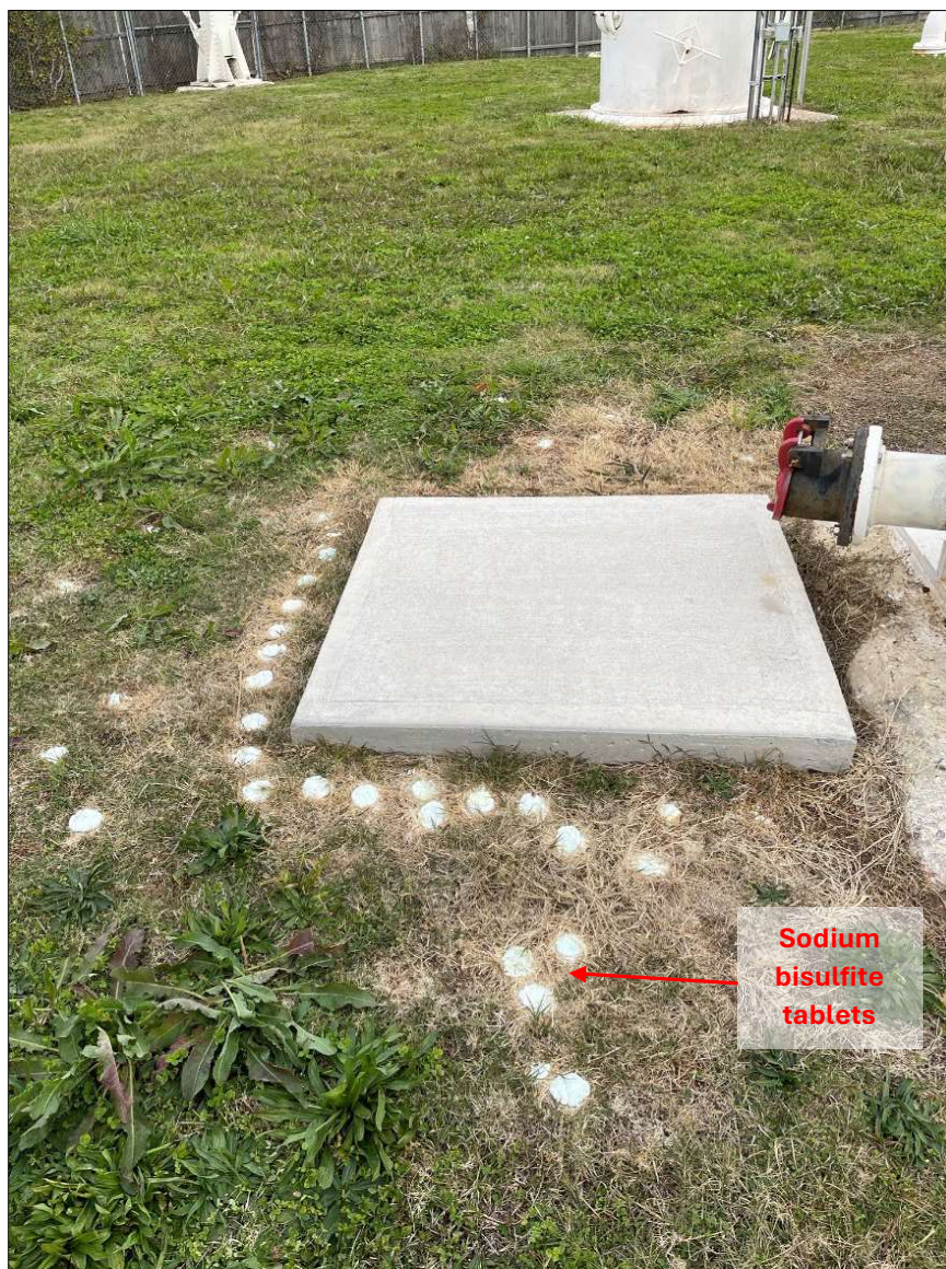
Photograph 17. A Tower North IMG_3109.jpeg
