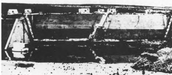
FIGURE 7. Disposal in concrete silos.
