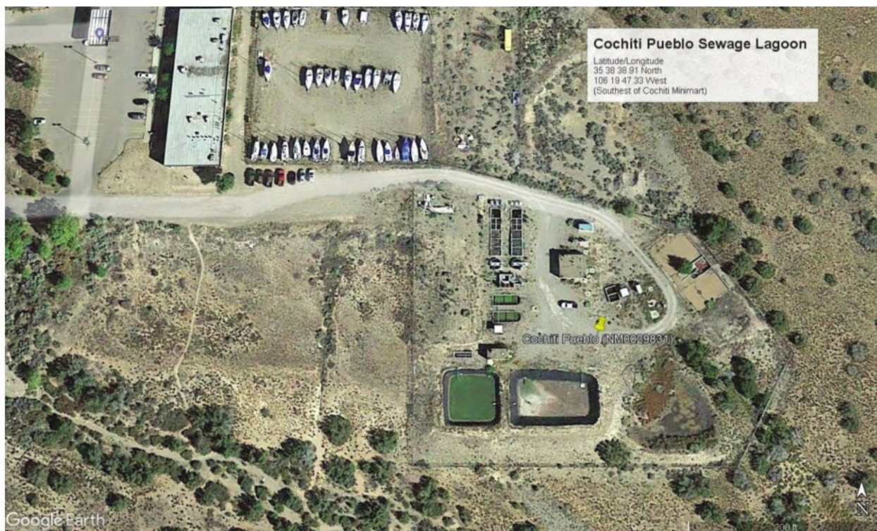
Aerial Image #1: Overall view of the Cochiti Pueblo Sewage Lagoon location. Aerial from Google Earth Maps.
