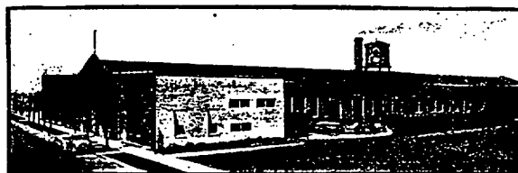
USG Steel Products Plant at Chicago
