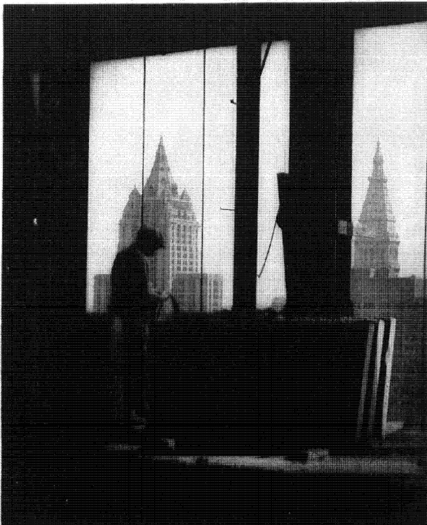
A stone worker on New York's newest skyscraper, high up in the air. The New York Life and Metropolitan Life Insurance Company buildings are seen in the background.
