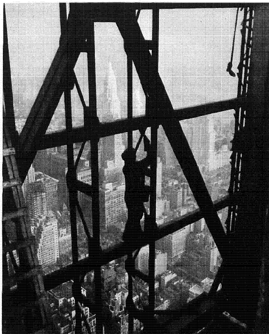
This painter, 1,248 feet above ground, is putting the finishing touches on the framework of the mooring mast that tops the Empire State Building
