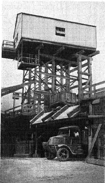
Speaking of headframes, here's one at Shaft 14-A, in Brooklyn, with a truck taking on a load of rock.
