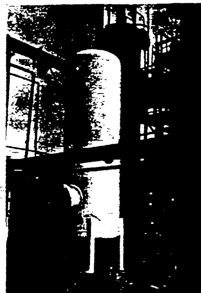
This sulphuric acid drying drum is protected with a paint system containing a red lead-alkyd primer coat and has withstood severe acid spillage and fume conditions for four and one-half years.
