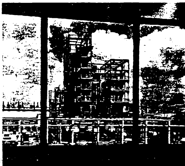
Operating plant structures for producing tetraethyl lead are also protected with a red lead anticorrosive-vinyl finish paint system. The system is performing well after three years of rigorous industrial exposure.
