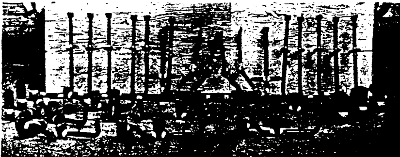
Below, some of the lead fixture connections, wastes and vents, installed in a low-rent project in Orange, Texas, and right, the lead and cast-iron roughing-in for back-to-back bathrooms in the project at Wynnewood, Pa.
