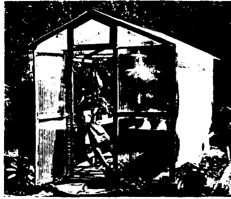
GREENHOUSES: Many plastics, including glass-reinforced polyester (above), acrylic, polycarbonate, films, etc., are used in glazing.
