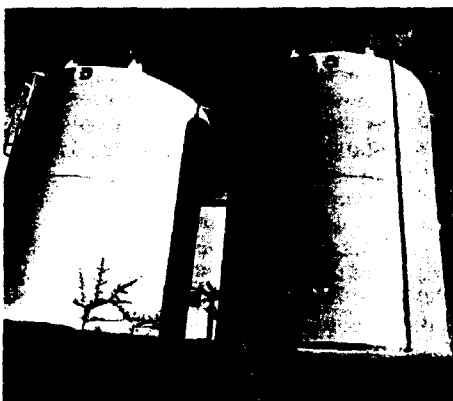
STORAGE TANKS: Huge corrosion-resistant reinforced plastics tanks for chemicals can be produced at half the price of stainless steel.
