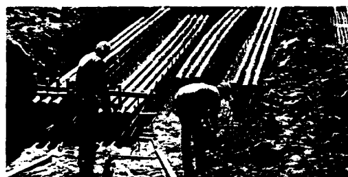
CONDUIT: Major part of the pipe market is serviced by lightweight polyethylene conduit (above, for a gas and electric power plant).
