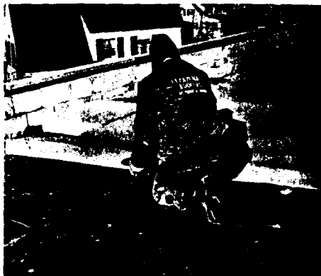
BUILDING INSULATION: Urethane foam (above) and expanded styrene foam roof insulation are builder's newest tools in conserving energy.
