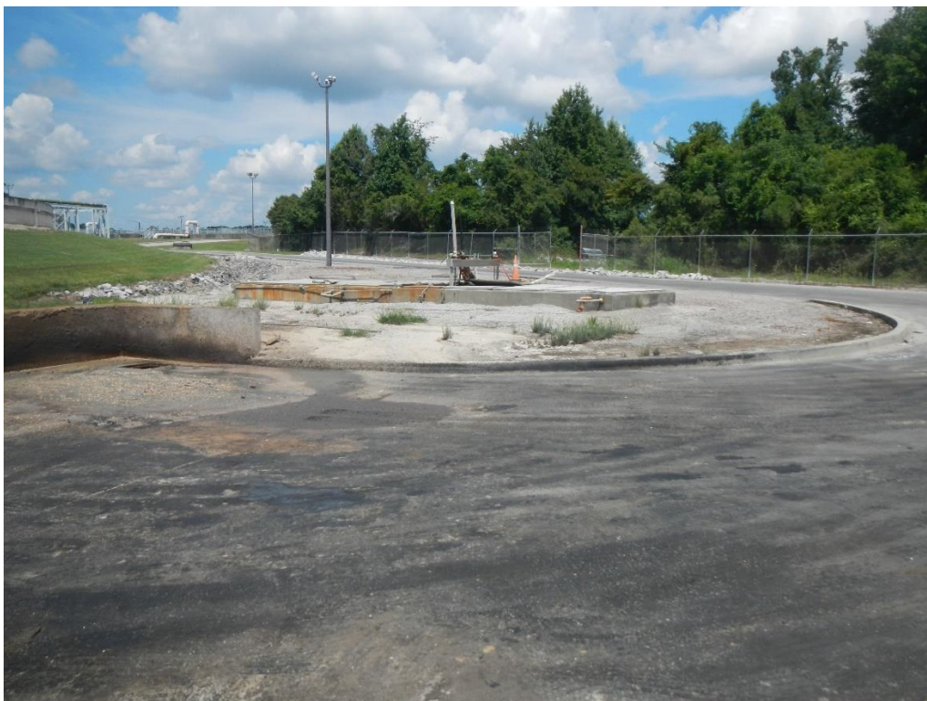
Photo 1: Headworks of facility
