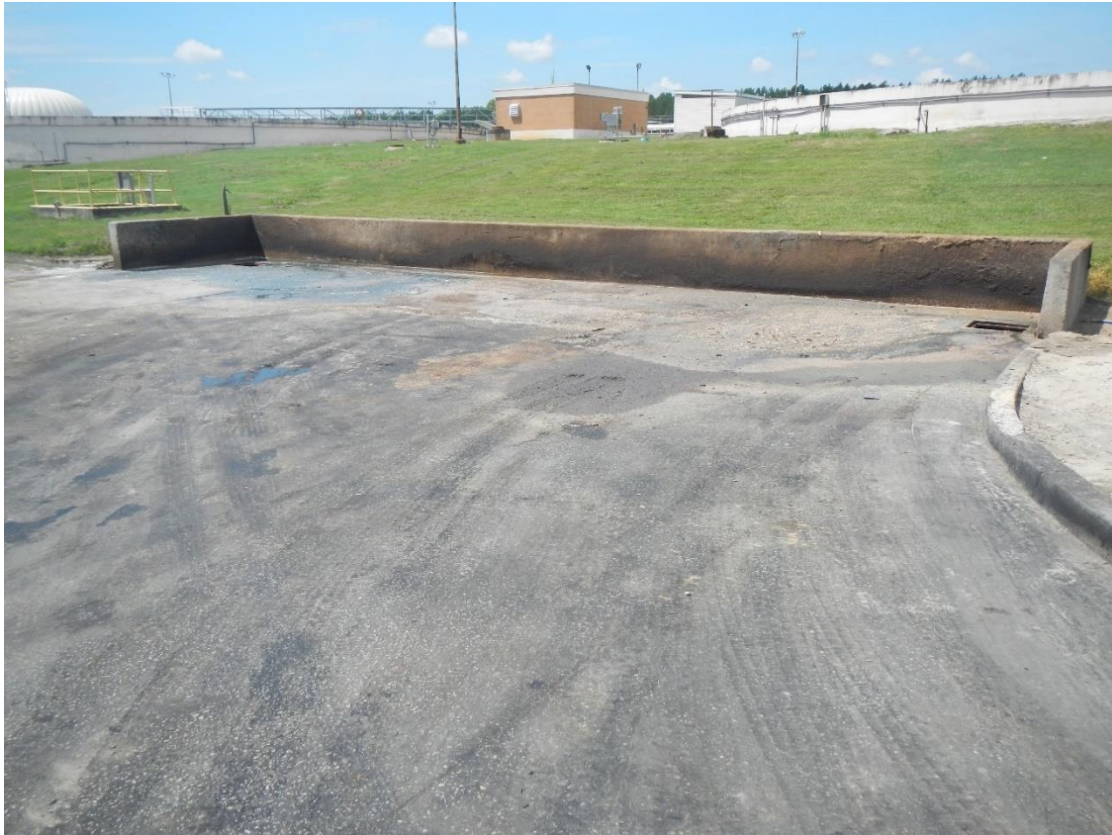
Photo 3: Septic hauler receiving area.
