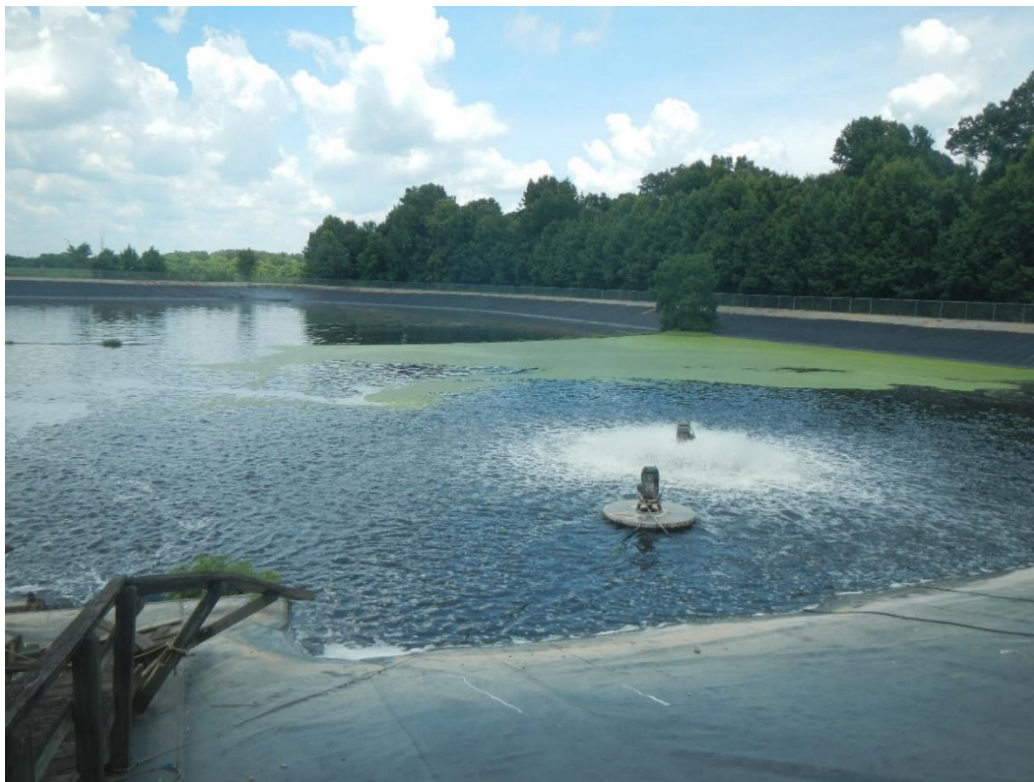
Photo 10: Constructed wetlands final aeration basin.
