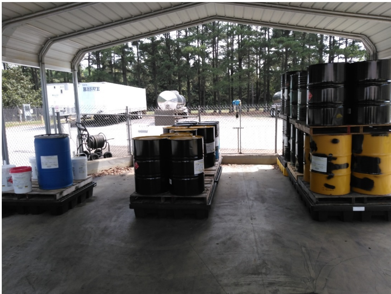
Photograph 7: General view of the containers in the hazardous waste storage pad.
