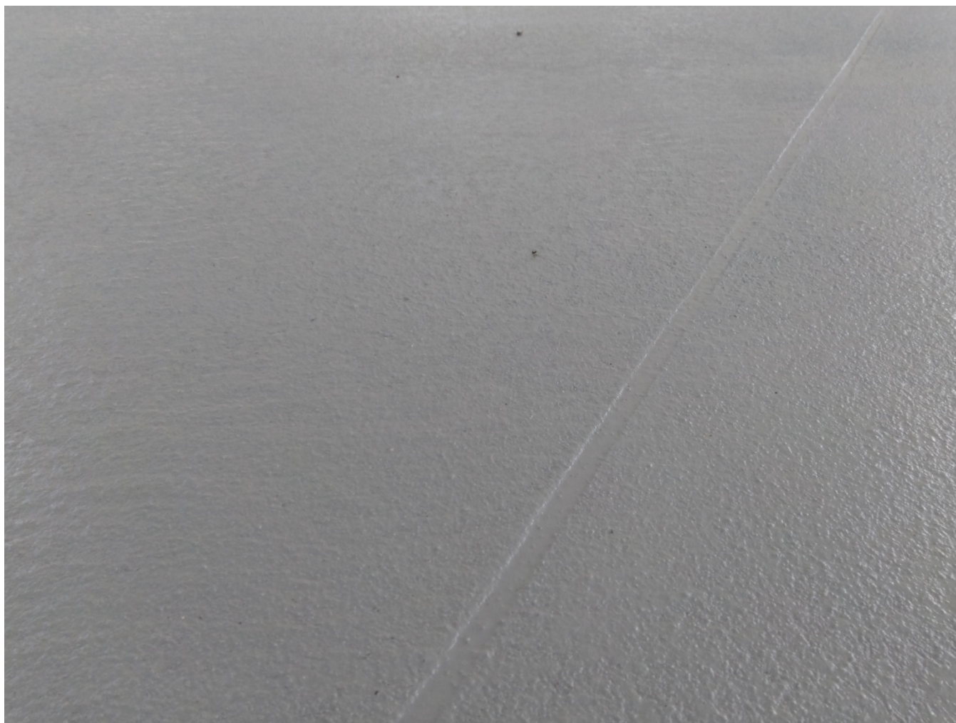
Photograph 9: View of the hazardous waste storage pad's floor to document coating with sealant. Milliken took the photograph on June 21, 2021.
