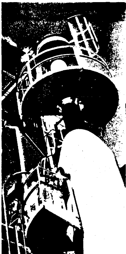
At Sauget, Ill., plant, $500,000 incinerator will destroy waste PCB at 3,000 F.
